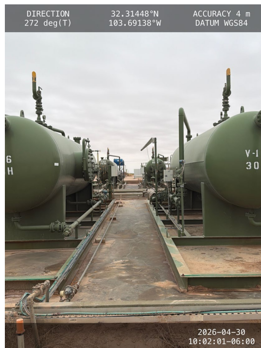
Photo 12 View of the central area of the secondary containment towards west.
