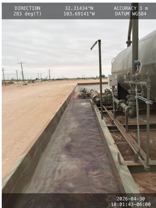
Photo 9 View of northwest corner of containment.
