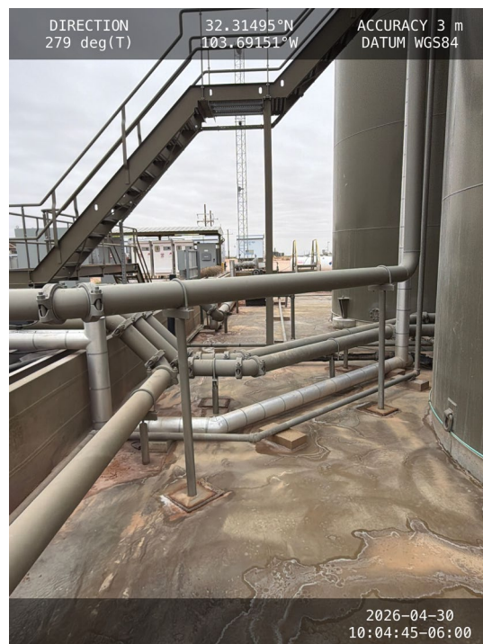
Photo 10 View of containment towards west.
