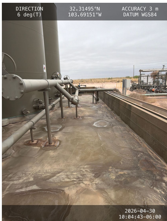
Photo 11 View of containment towards north.
