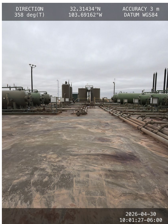
Photo 13 View of central containment towards north.
