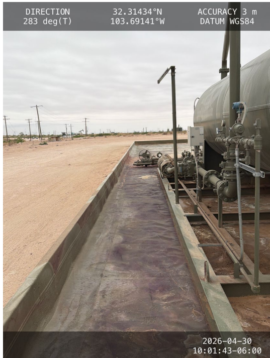
Photo 9 View of northwest corner of containment.
