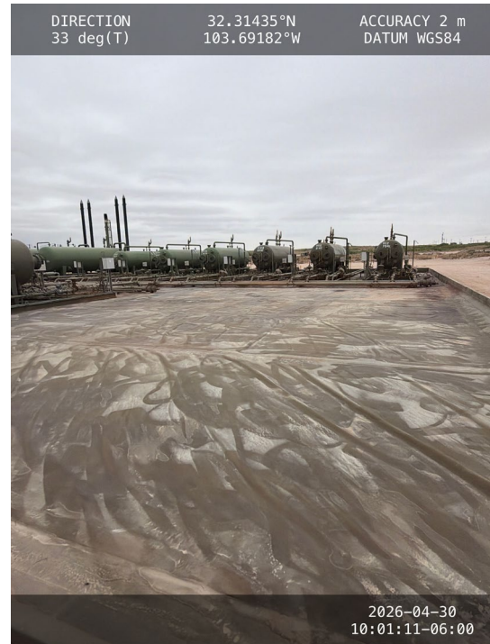
Photo 2 View of north-northeast side of containment.
