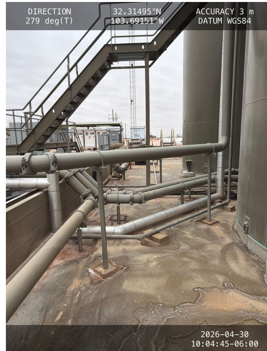
Photo 10 View of containment towards west.
