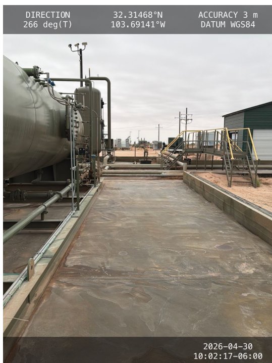
Photo 15 View of containment towards west.
