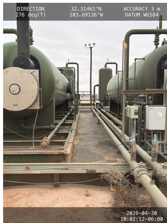
Photo 13 View of the secondary containment towards west.
