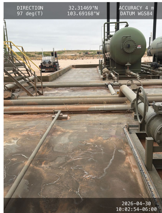
Photo 8 View of containment towards east.
