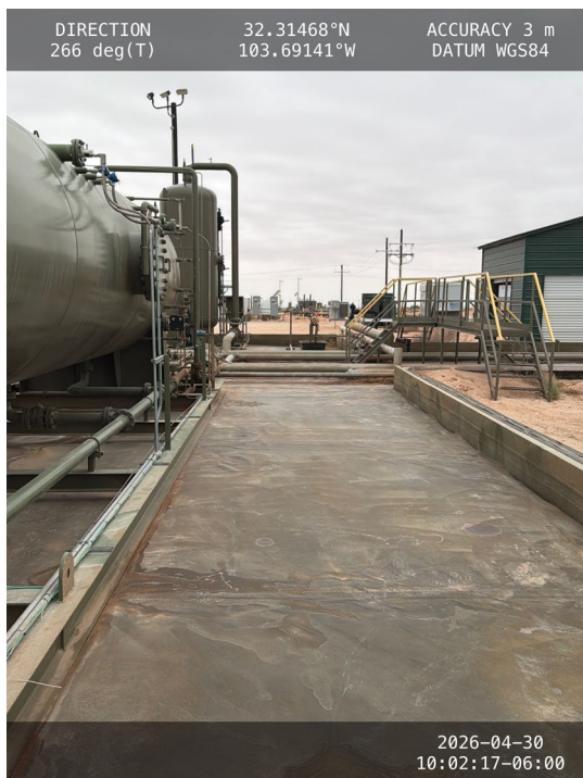
Photo 15 View of containment towards west.
