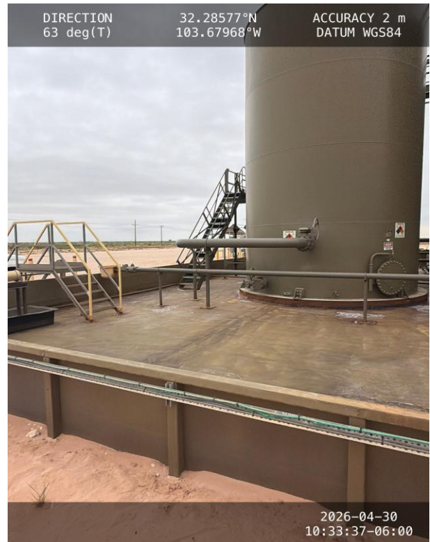
Photo 8 View of northwest corner of containment.
