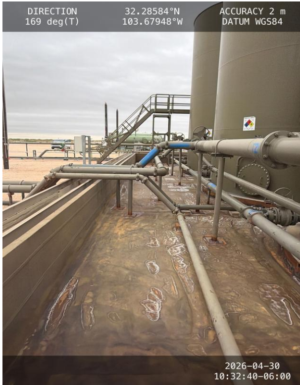
Photo 5 View of east side containment towards south.
