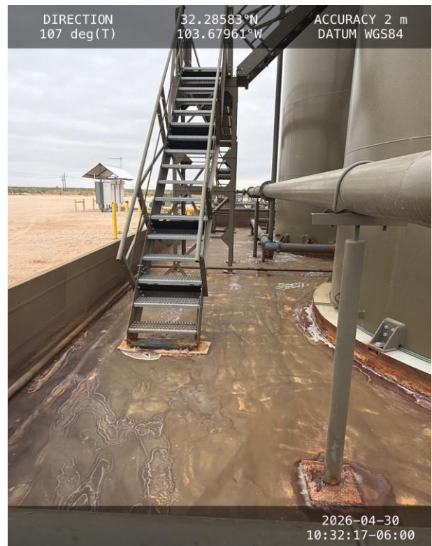
Photo 4 View of north side containment towards east.
