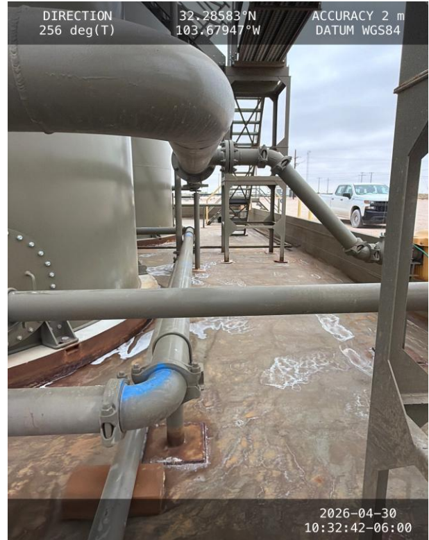
Photo 6 View of east side containment towards north.
