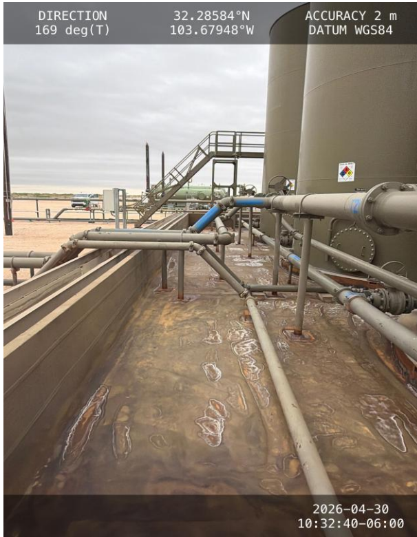
Photo 5 View of east side containment towards south.
