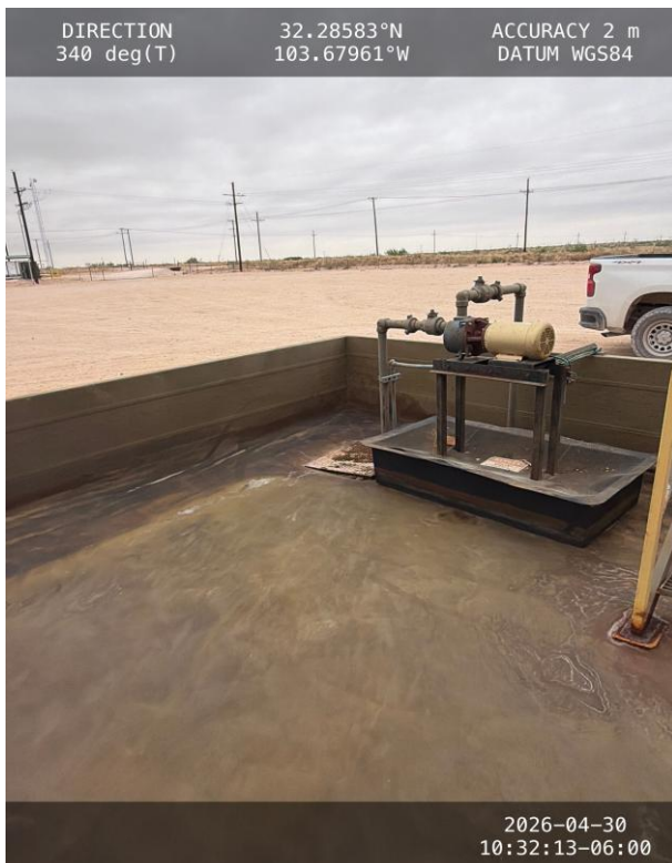
Photo 3 View of northwest corner of secondary containment.
