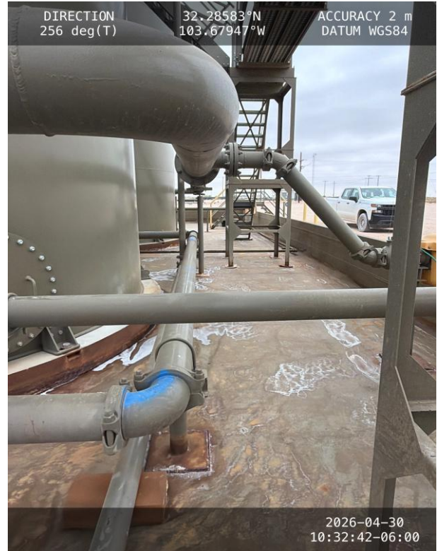
Photo 6 View of east side containment towards north.
