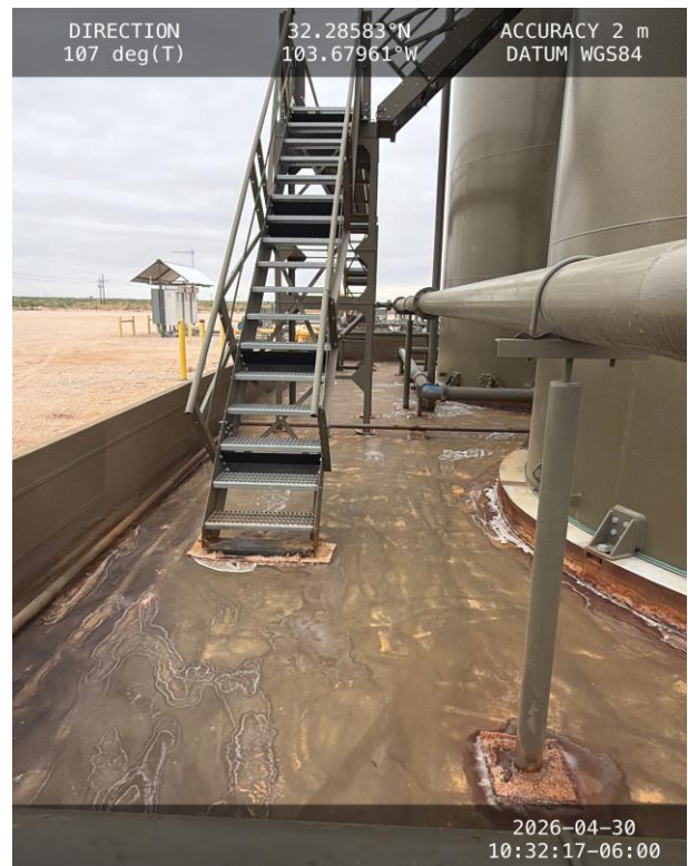
Photo 4 View of north side containment towards east.
