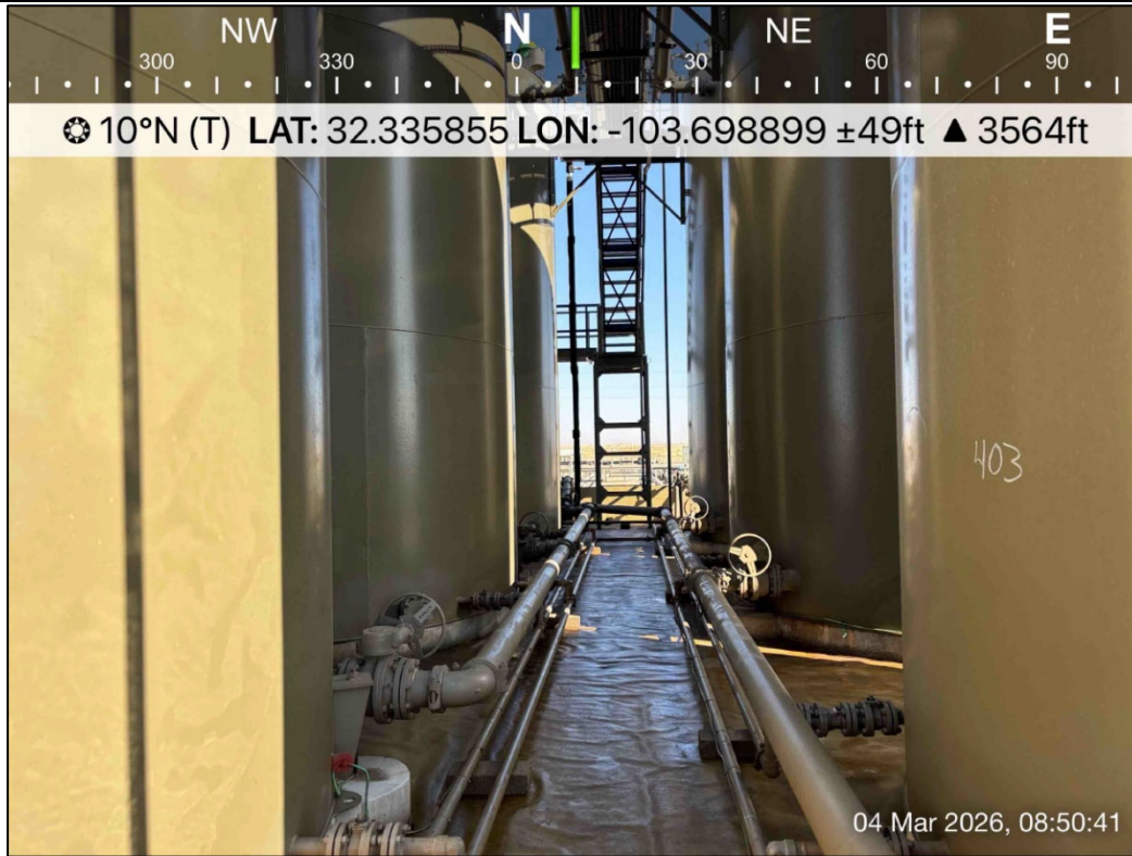
PHOTO 9: Northern view during liner inspection activities. 3/4/2026
