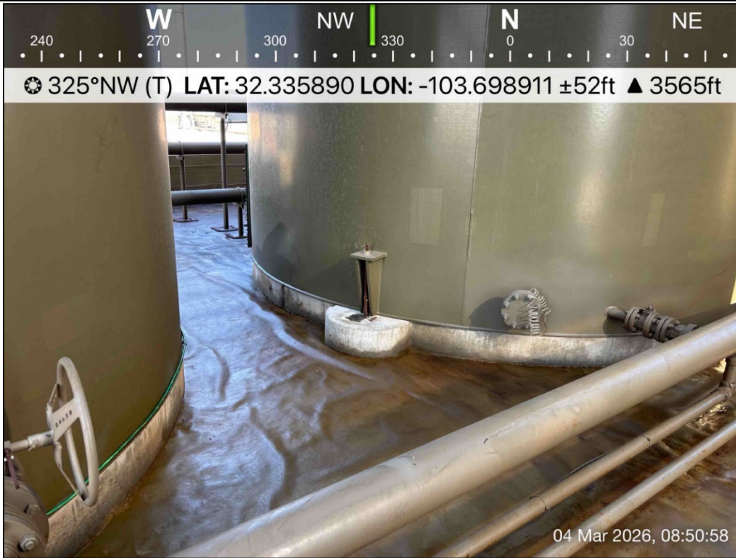
PHOTO 11: Northwestern view during liner inspection activities. 3/4/2026
