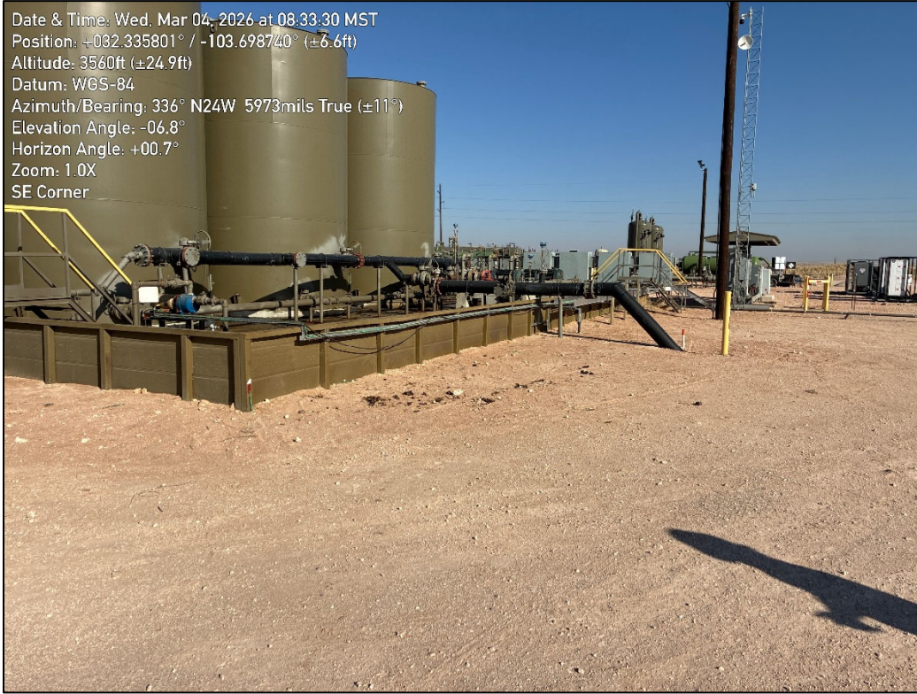
PHOTO 15: Northwestern view outside of containment during liner inspection activities. 3/4/2026
