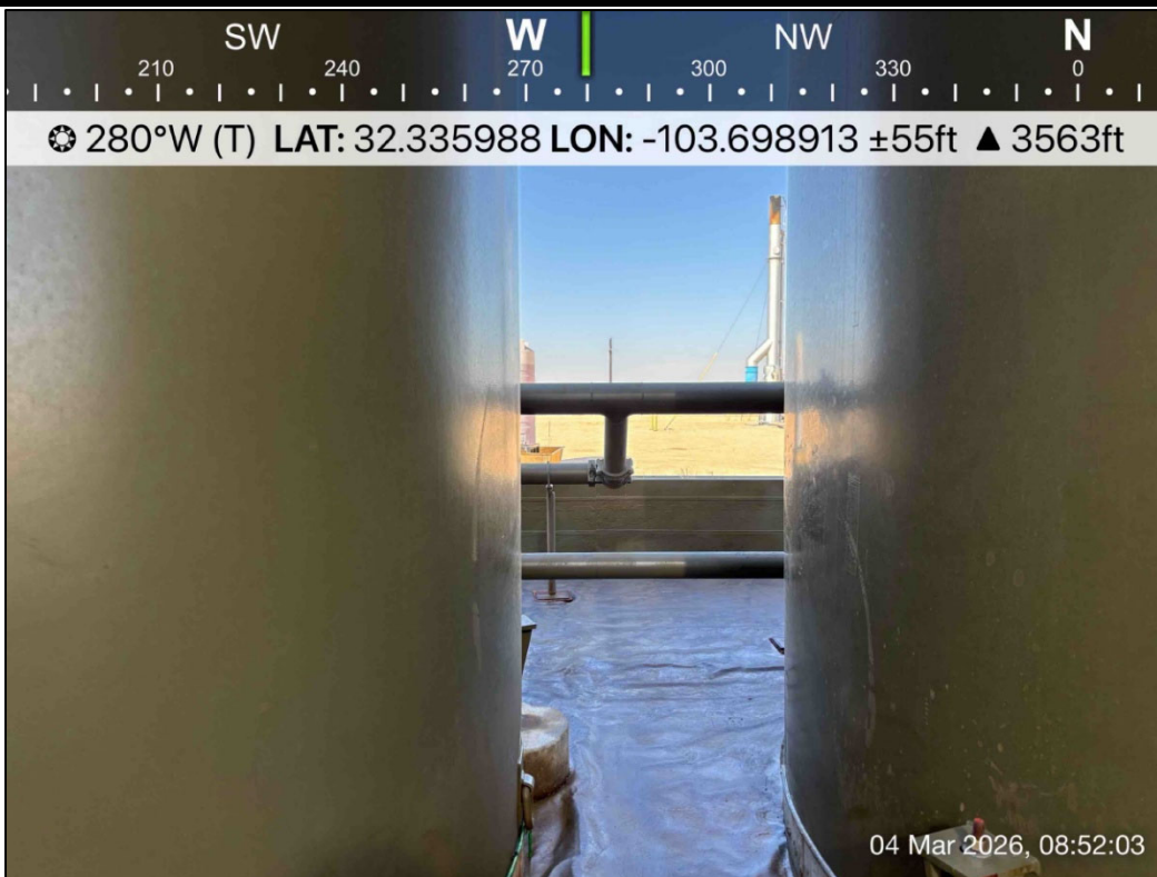
PHOTO 12: Western view during liner inspection activities. 3/4/2026
