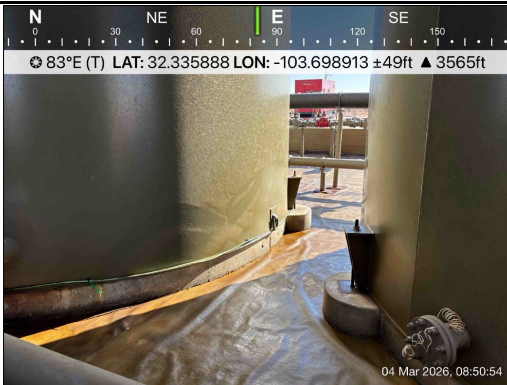
PHOTO 10: Northeastern view during liner inspection activities. 3/4/2026
