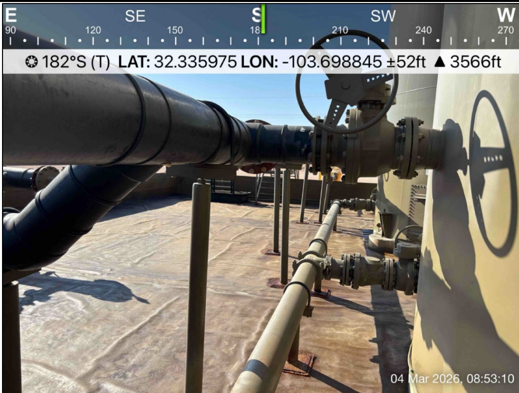
PHOTO 14: Southern view during liner inspection activities. 3/4/2026
