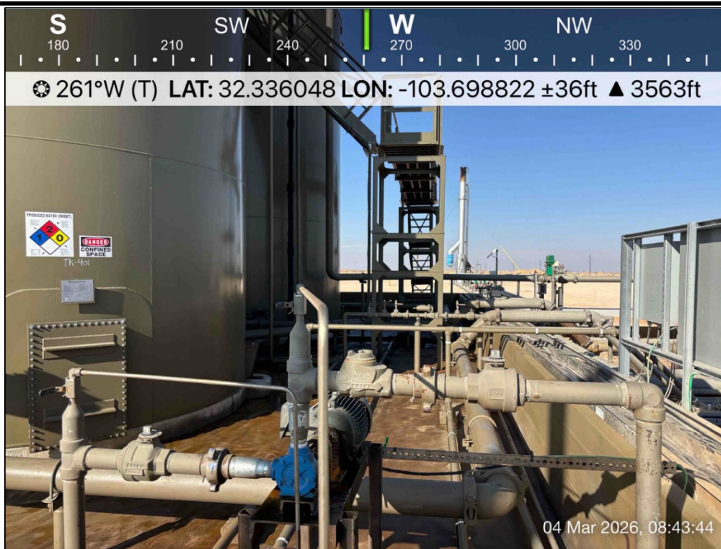
PHOTO 5: Western view during liner inspection activities. 3/4/2026
