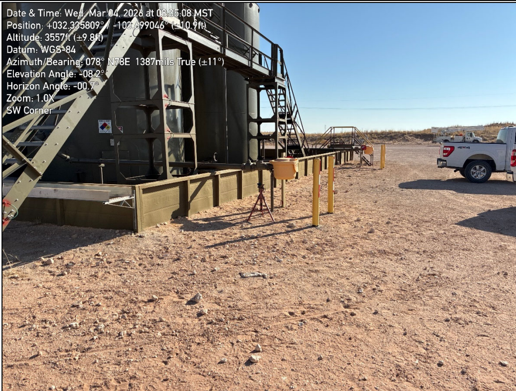
PHOTO 18: Northeastern view outside of containment during liner inspection activities. 3/4/2026
