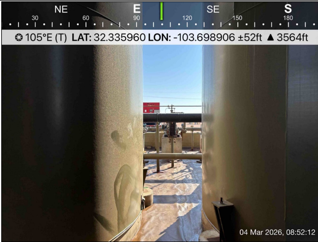
PHOTO 13: Eastern view during liner inspection activities. 3/4/2026
