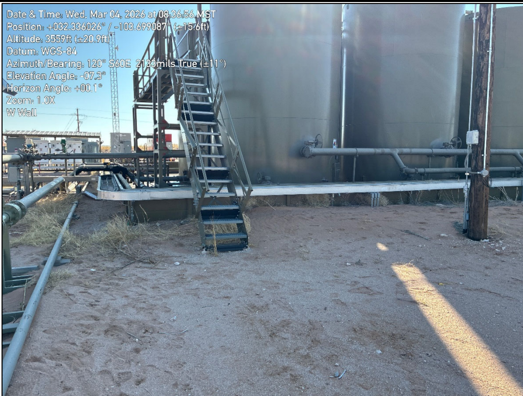
PHOTO 20: Southeastern view outside of containment during liner inspection activities. 3/4/2026
