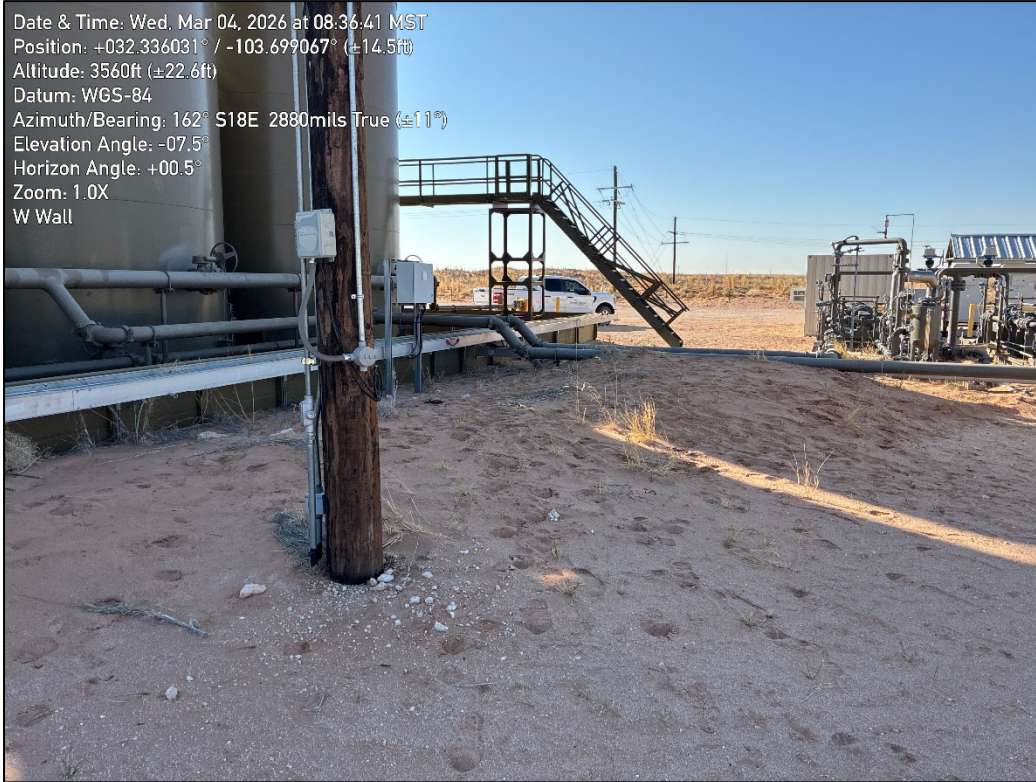
PHOTO 19: Southeastern view outside of containment during liner inspection activities. 3/4/2026
