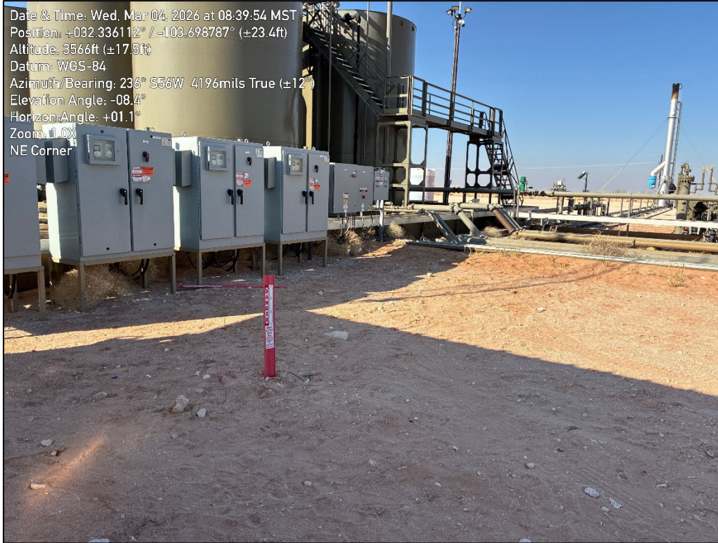
PHOTO 23: Southwestern view outside of containment during liner inspection activities. 3/4/2026
