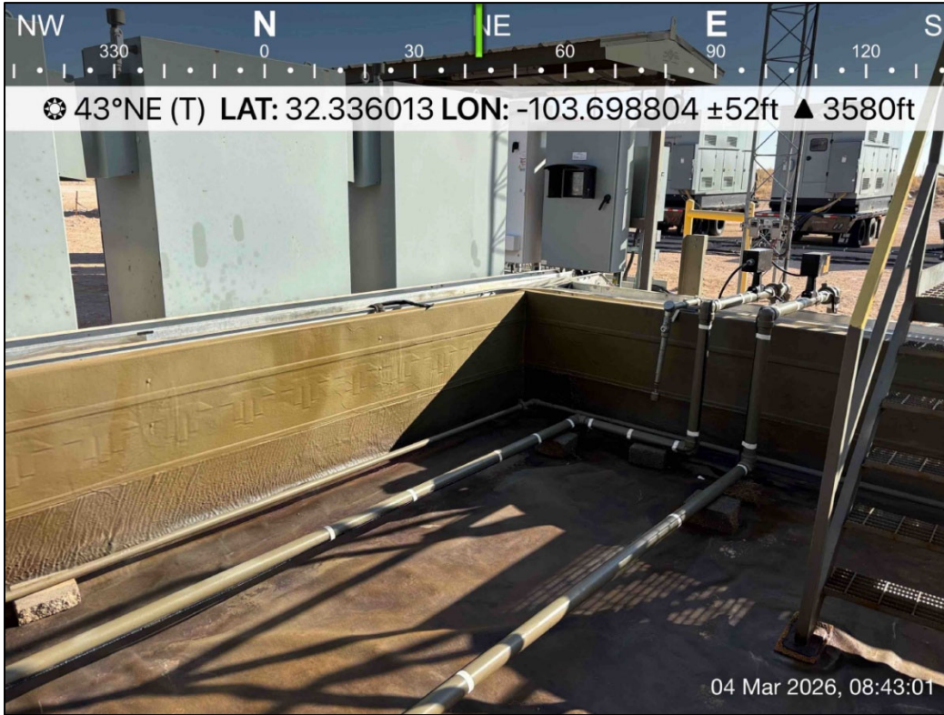
PHOTO 3: Northeastern view during liner inspection activities. 3/4/2026
