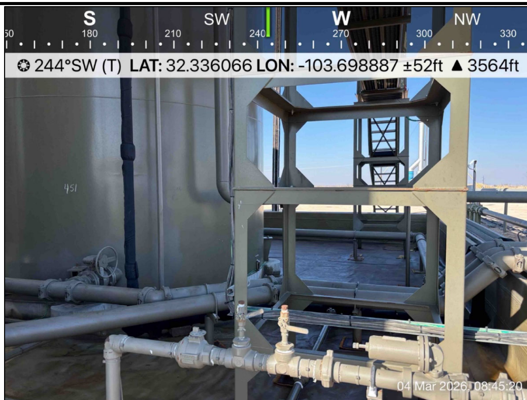
PHOTO 6: Southwestern view during liner inspection activities. 3/4/2026
