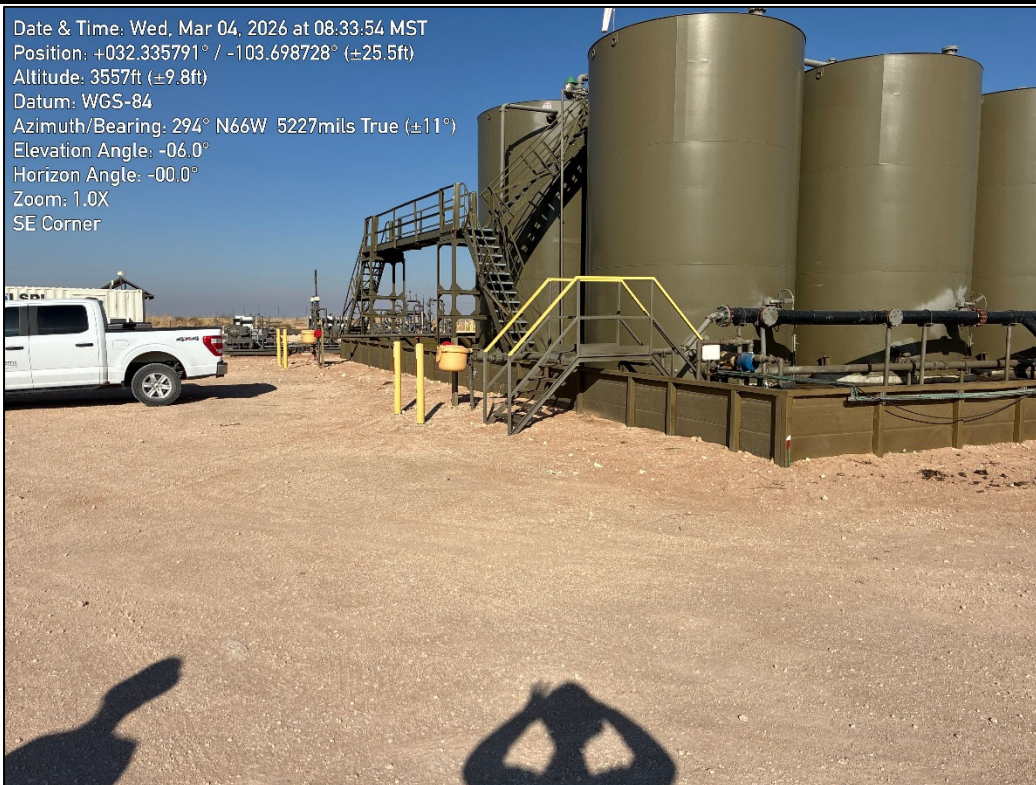
PHOTO 16: Northwestern view outside of containment during liner inspection activities. 3/4/2026
