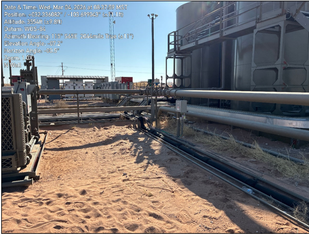
PHOTO 21: Southeastern view outside of containment during liner inspection activities. 3/4/2026
