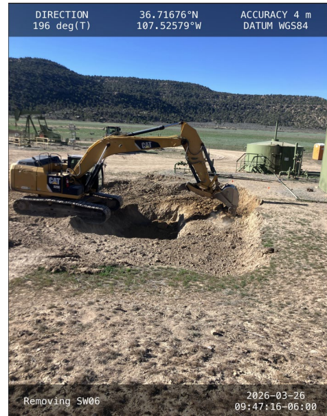
Photograph: 4 Date: 3/26/2026 Description: Removing SW06, Collecting SW07 View: South
