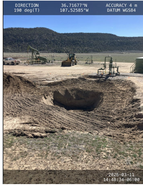
Photograph: 2 Date: 3/11/2026 Description: Northwest side of Excavation Day 2 View: South
