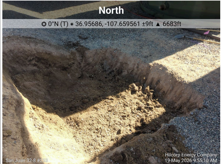
Photograph: 8 Description: Final excavation extent. View: North
