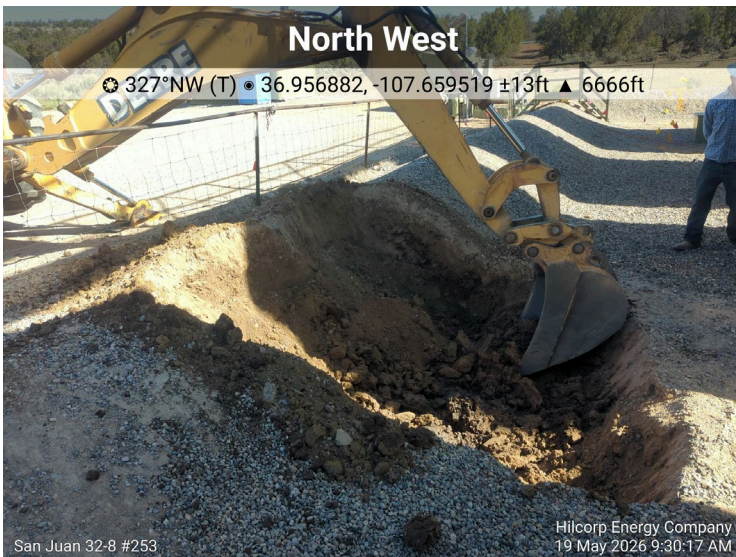
Photograph: 7 Description: Additional excavation activities View: Northwest
