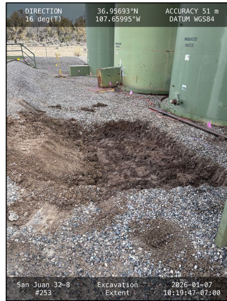
Photograph: 6 Description: Initial Excavation Extent View: West
