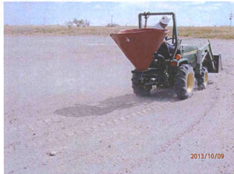
Seeding soil, facing southeast 10/9/13
