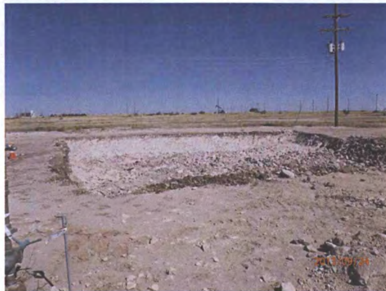
Excavating on lease pad completed, facing north 9/24/13
