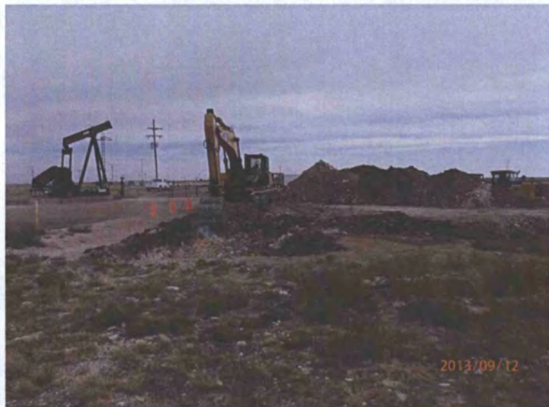
Excavating around lease pad, facing east 9/12/13
