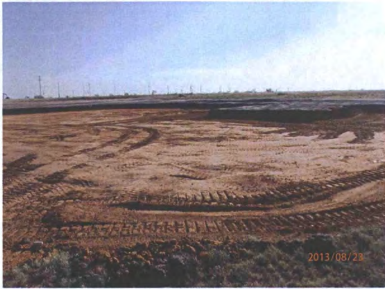
Clay liner installed in east excavation at 4 ft bgs, facing east-northeast 8/23/13
