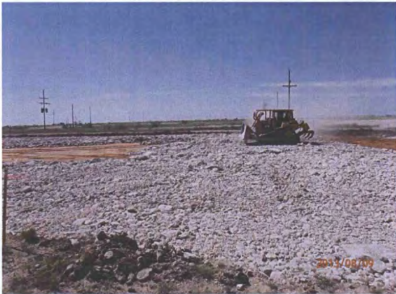
Placing 1 foot of rock over clay, facing south 8/9/13
