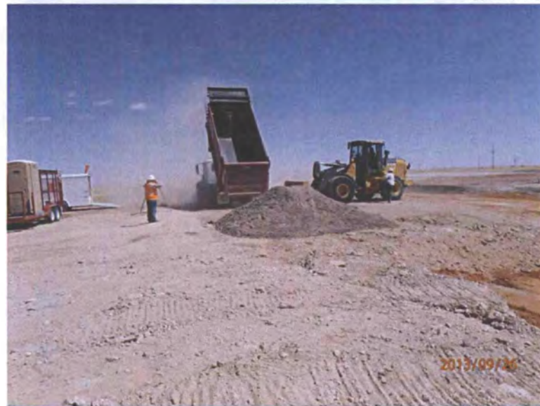
Importing soil, facing east 9/26/13
