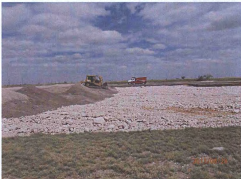
Placing topsoil over east excavation, facing east 8/28/13
