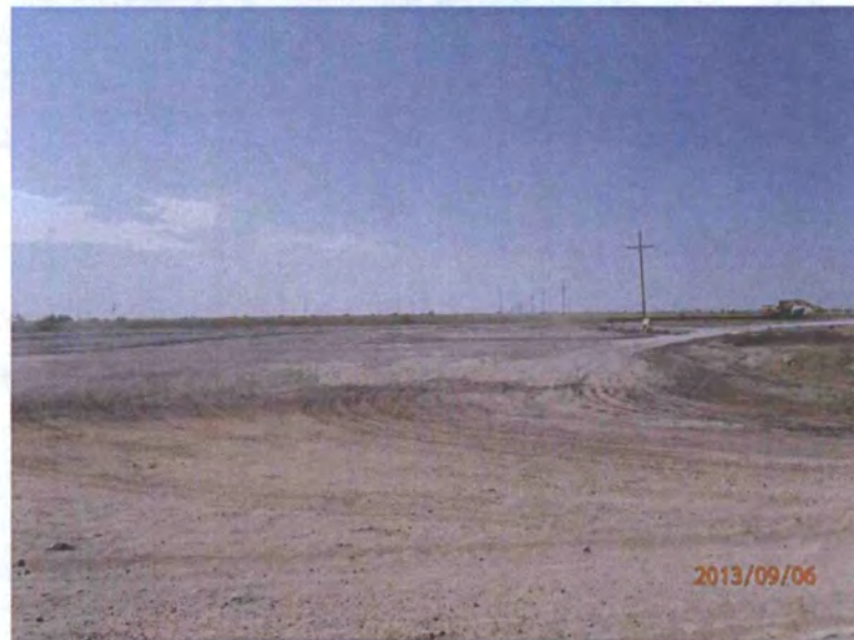
East end excavation completed, facing south 9/6/13
