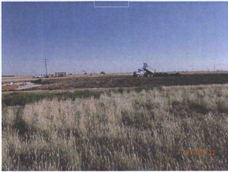
Importing topsoil, facing north 8/22/13
