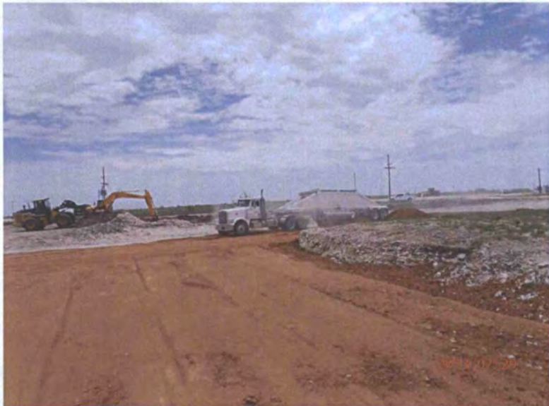
Importing clay, facing south
