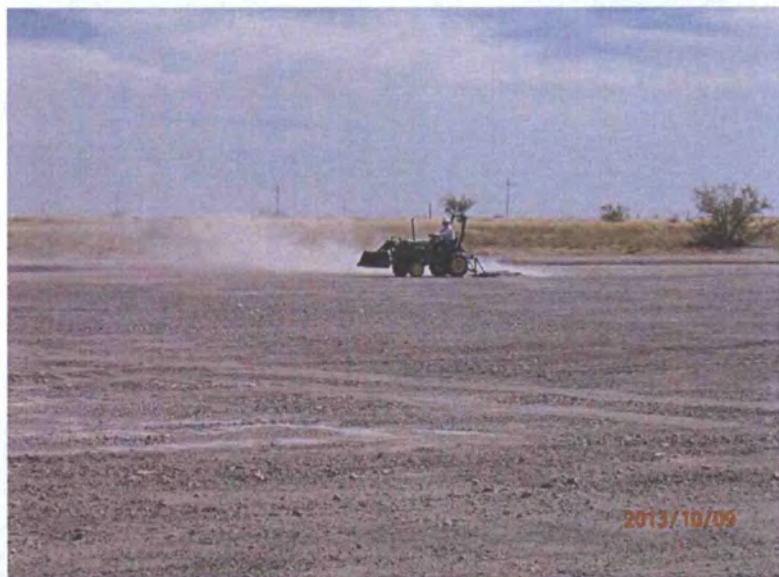
Ripping soil prior to seeding, facing north 10/9/13
