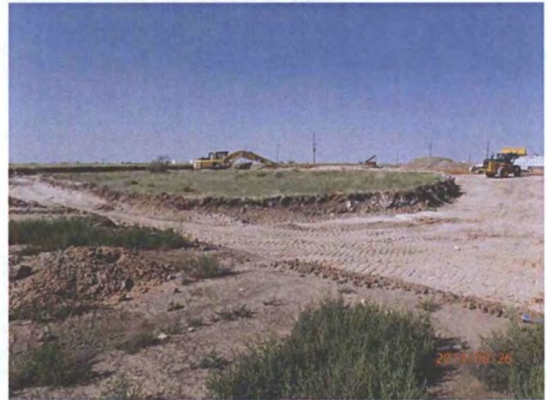
Completed middle excavation, facing southwest 8/26/13
