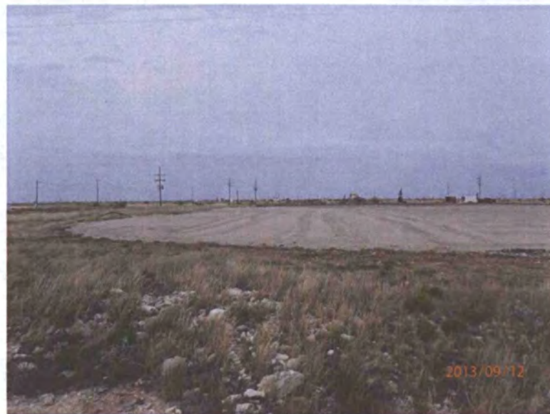
Middle excavation completed, facing west 9/12/13
