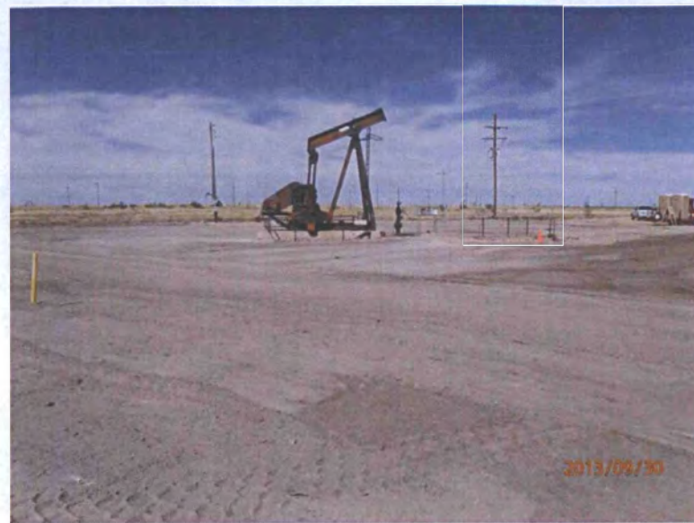
Lease pad excavation completed, facing north 9/30/13
