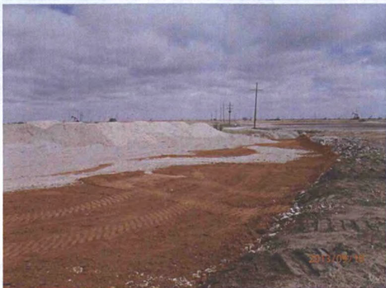
Backfilling middle excavation, facing north 9/10/13
