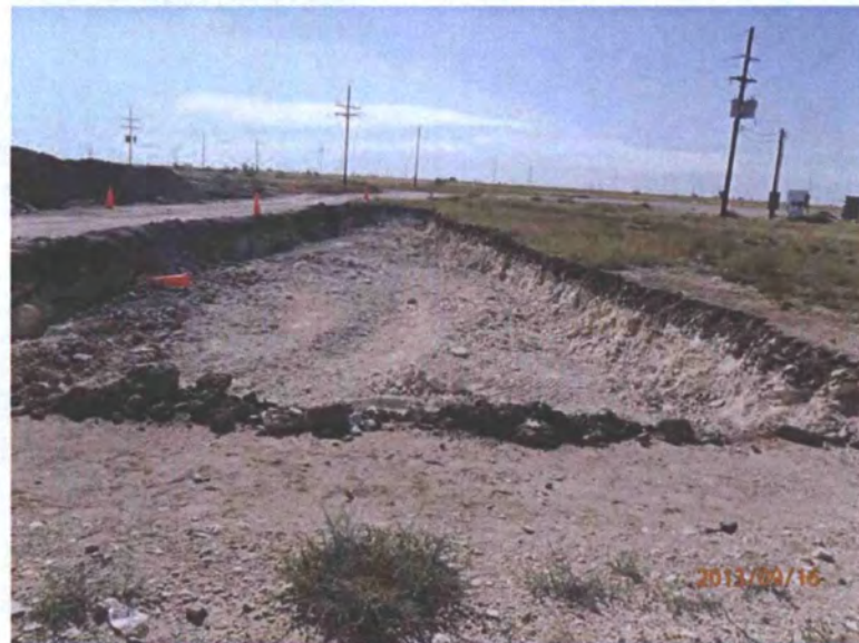
Excavation around lease pad completed, facing south 9/16/13
