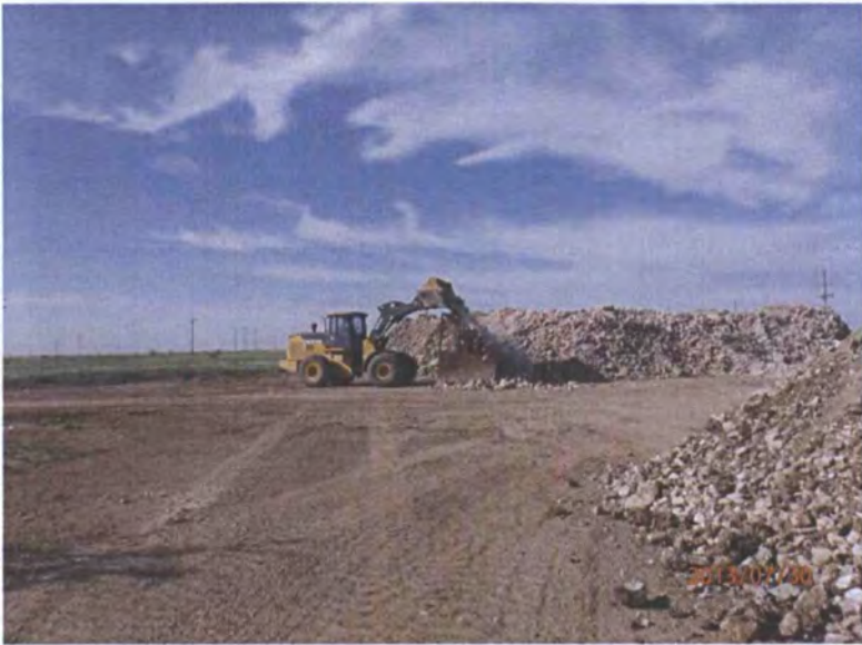
Screening rock from sand, facing west 7/30/2013
