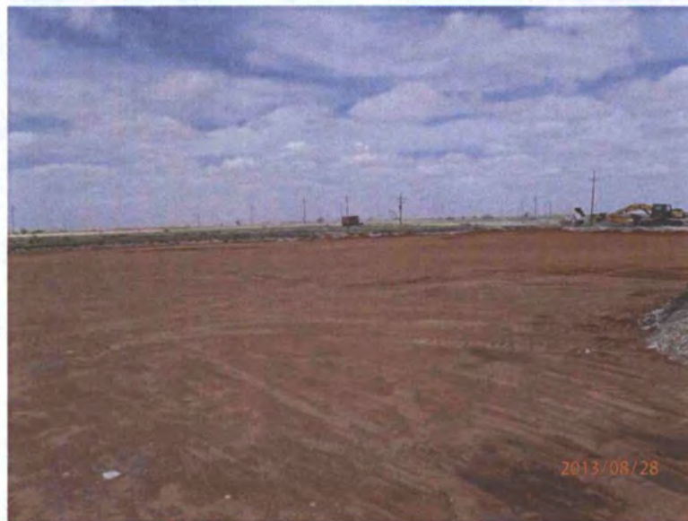
Completed clay liner in middle excavation, facing northeast 8/28/13
