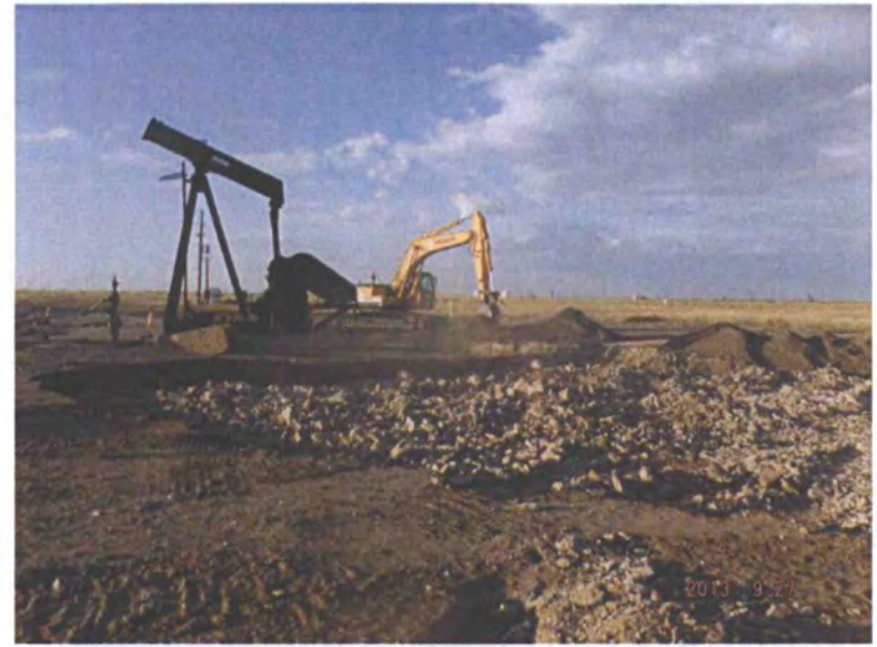
Installed rock layer on pad, facing southwest
