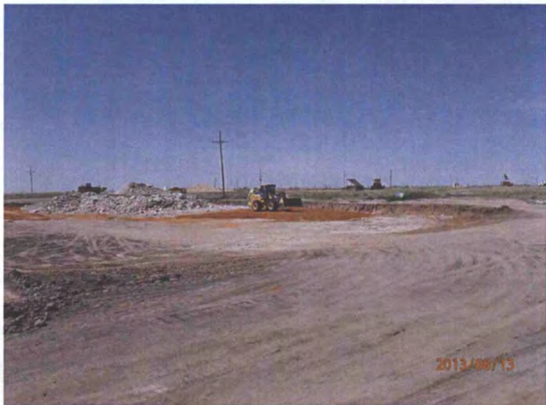
Installing clay liner on east side, facing SW 8/13/13
