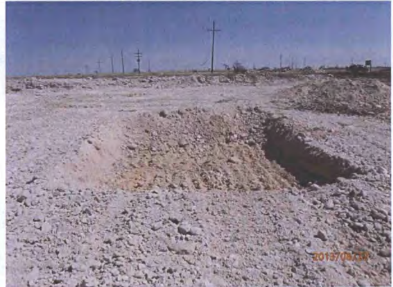
SB-22 excavation completed, facing northeast 8/22/13
