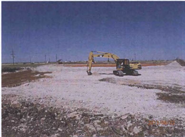
Excavating SB-22 another foot, facing west 8/22/13
