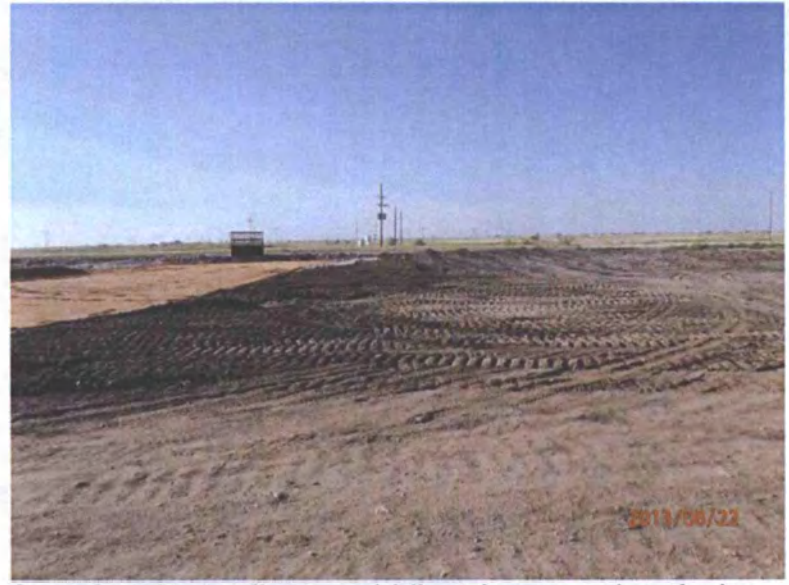
Completed topsoil over middle 4 ft excavation, facing south 8/22/13
