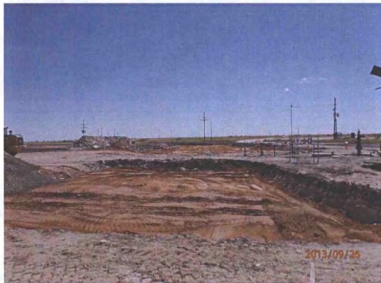
Clay liner installed in pad excavations, facing south 9/26/13
