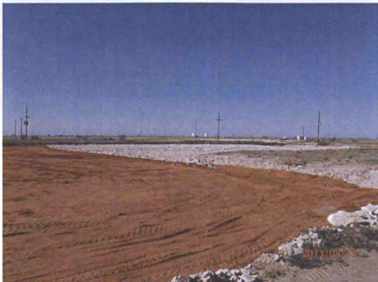
3 ft section with clay and 4 ft section with rock overlay, facing southwest 8/13/13
