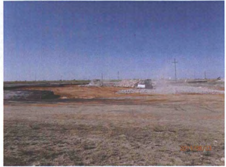
Installing 1 ft of rock over clay in east excavation, facing south 8/23/13
