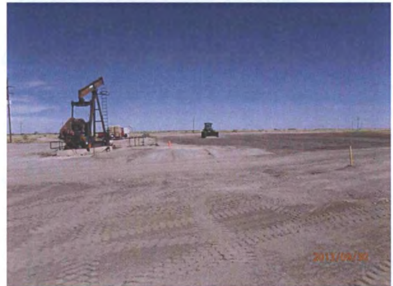
Back-dragging middle excavation, facing east
