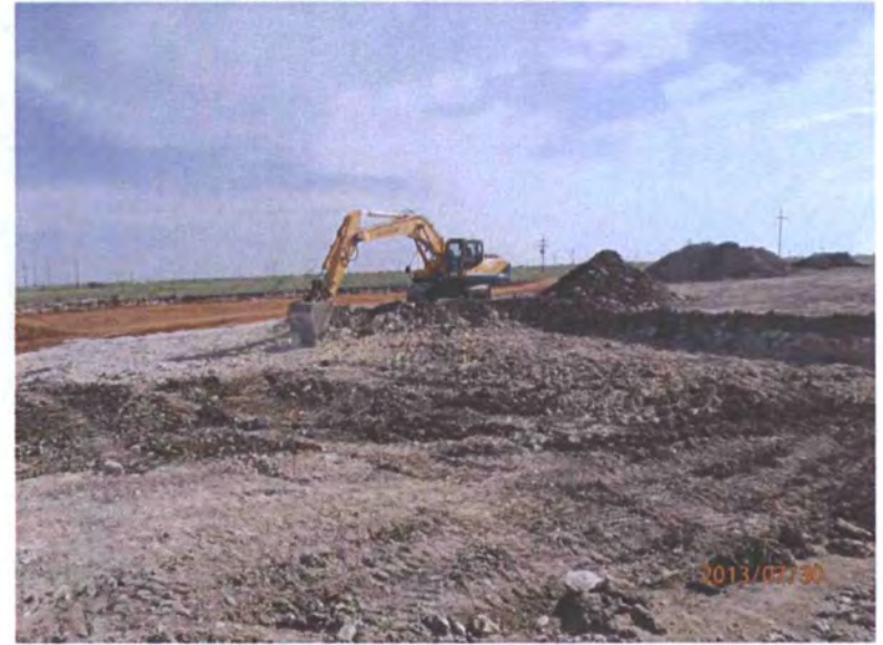
Continuing excavation, facing north 7/30/13
