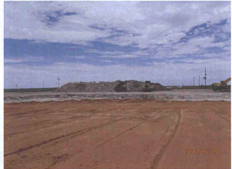
Clay liner, facing south
