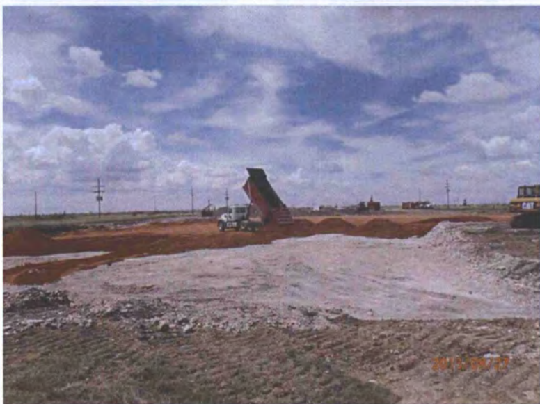
Installing clay liner in middle excavation, facing west 8/27/13
