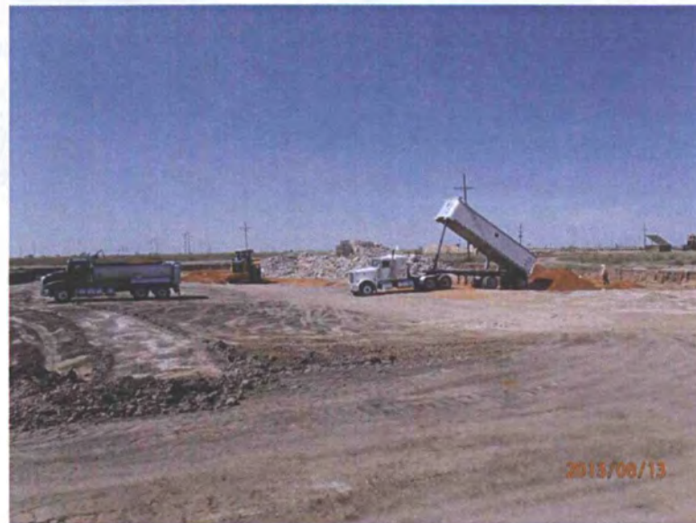
Importing clay and installing liner on east side excavation, facing southwest 8/13/13
