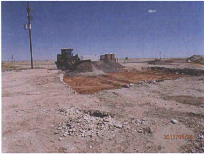
Backfilling lease pad, facing east
