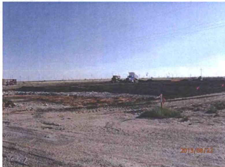
Installing topsoil over middle excavation, facing east 8/22/13
