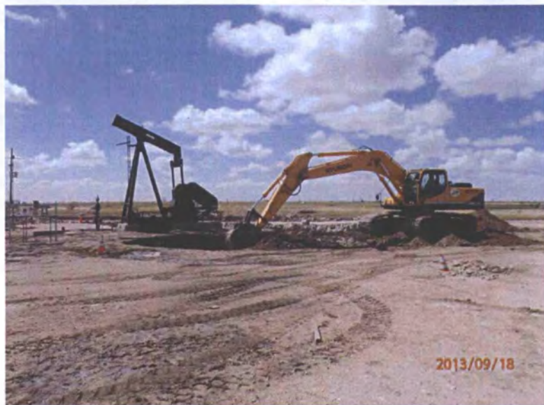
Excavating on lease pad, facing southwest 9/18/13
