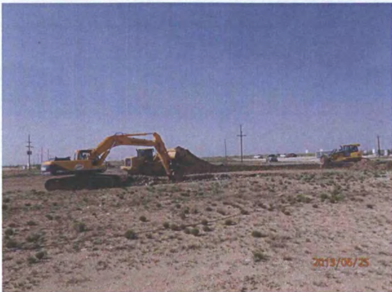
Excavating site, facing south
