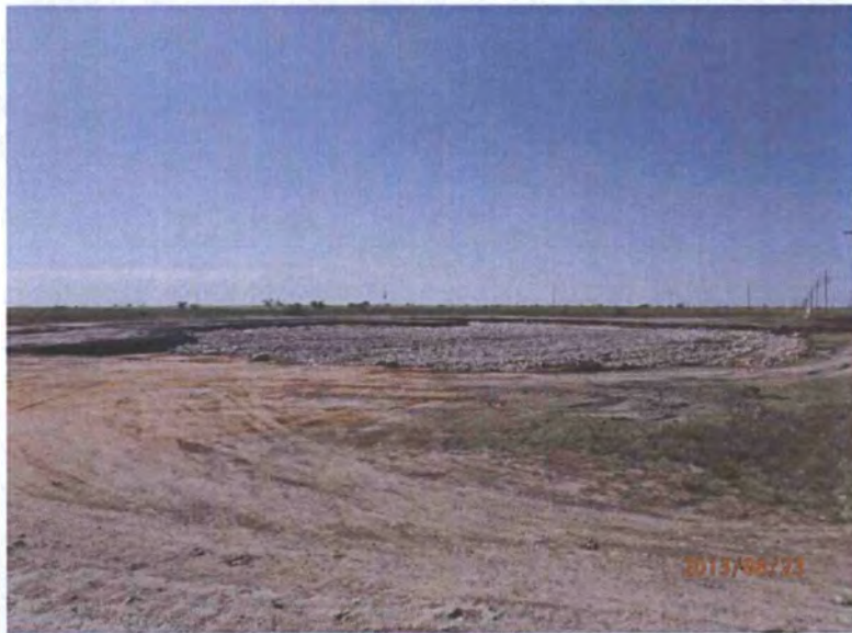
1 foot of rock over clay in east excavation completed, facing south 8/23/13
