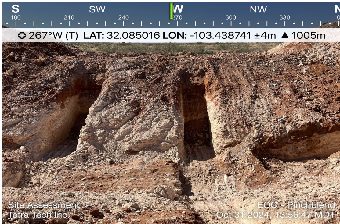
View of Remediation Activities – View West
