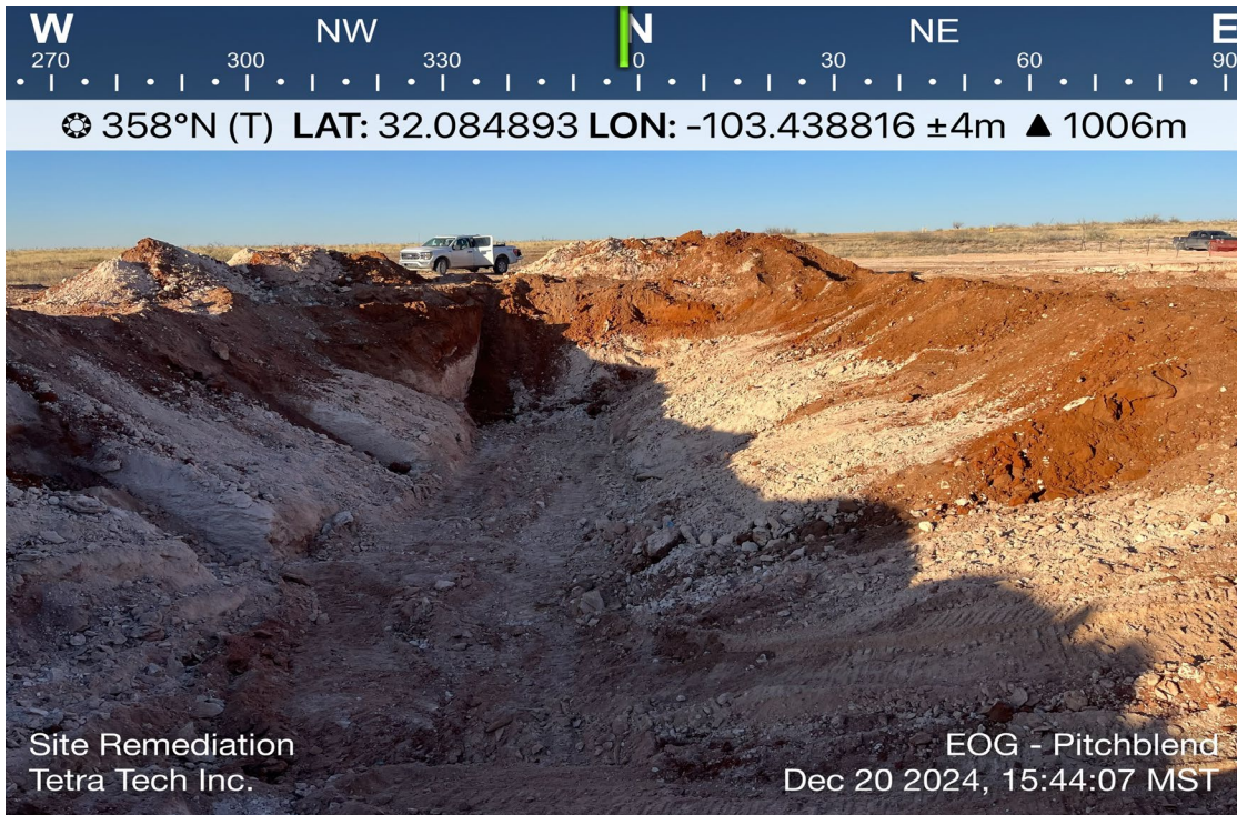
View of Remediation Activities – View North
