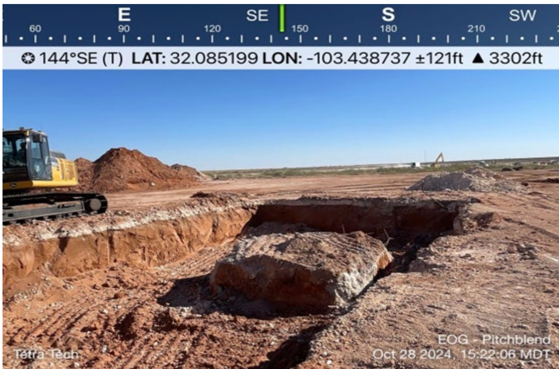
View of Remediation Activities – View Southeast
