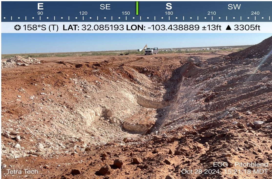
View of Remediation Activities – View South
