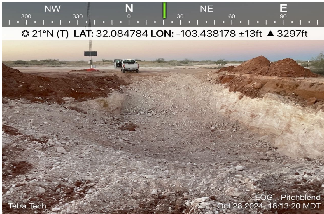
View of Remediation Activities – View North
