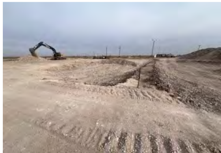
View to N of excavation.
