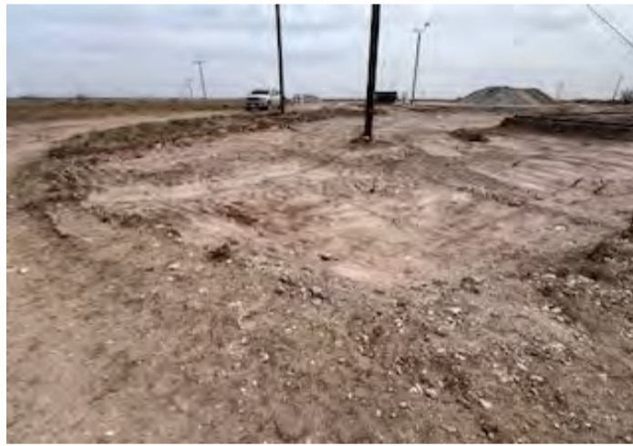
View to SE of N end of excavation.
