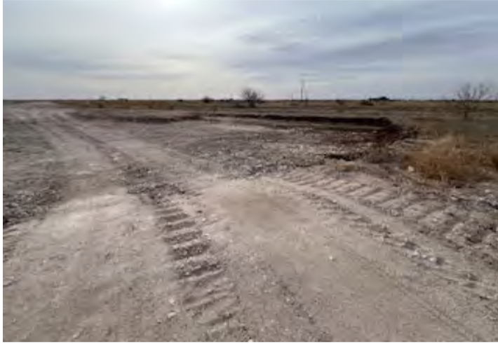
View to SE of S end of excavation.
