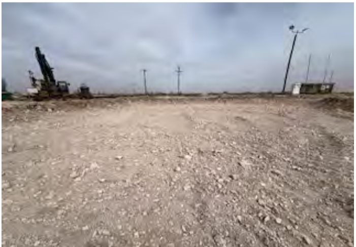
View to N of excavation.
