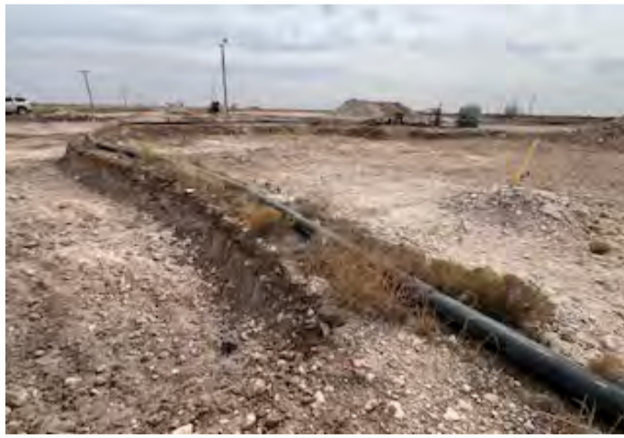
View to SE of excavation.
