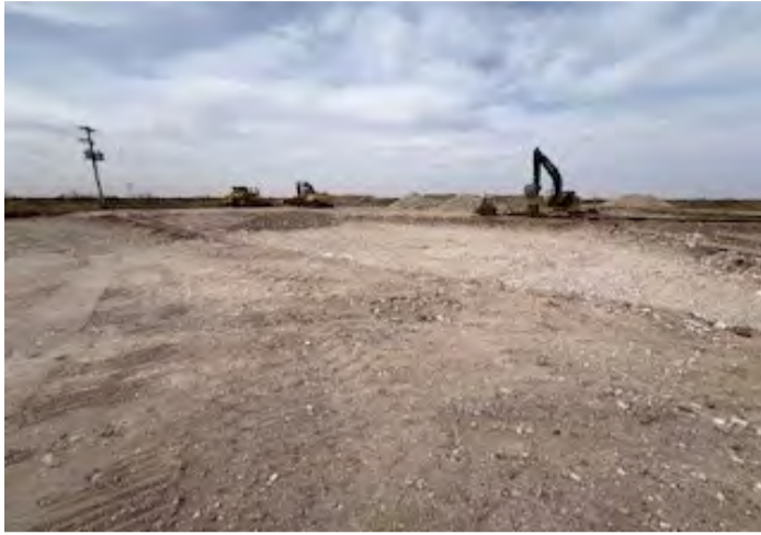
View to W of excavation.
