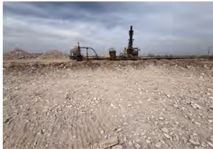
View to W of excavation, well, and pump.
