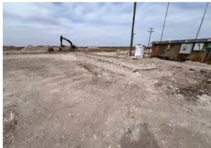
View to NW of excavation.
