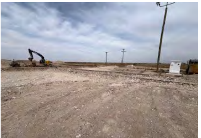
View to N of excavation.
