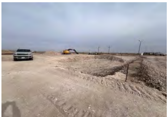
View to NW of excavation.
