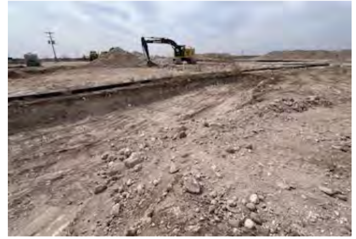
View to SW of excavation.
