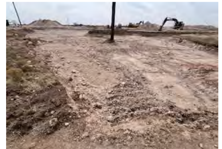
View to S of N end of excavation.
