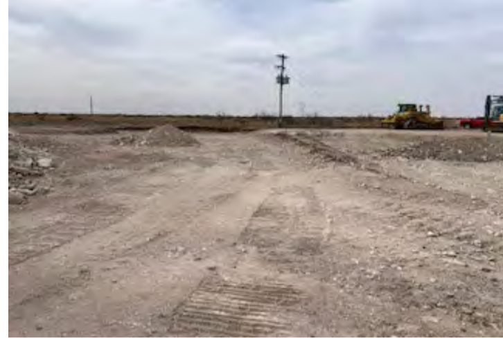
View to N of excavation.
