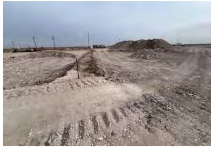
View to NE of excavation.
