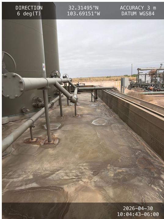
Photo 11 View of containment towards north.
