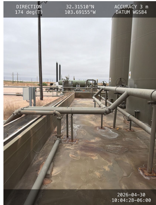
Photo 6 View of east side of containment towards south.
