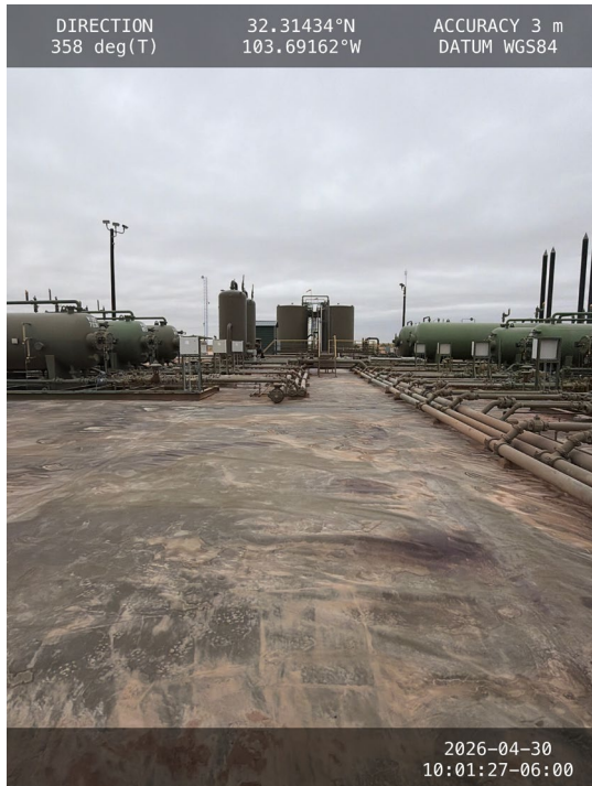
Photo 13 View of central containment towards north.
