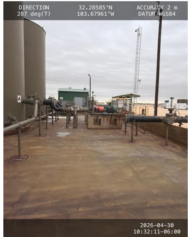
Photo 2 View of west side containment towards south.
