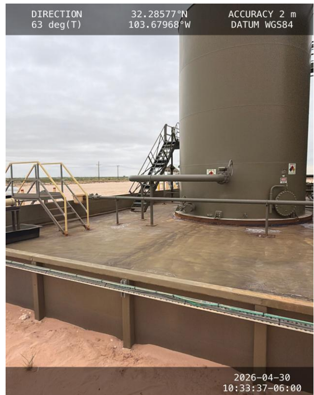
Photo 8 View of northwest corner of containment.
