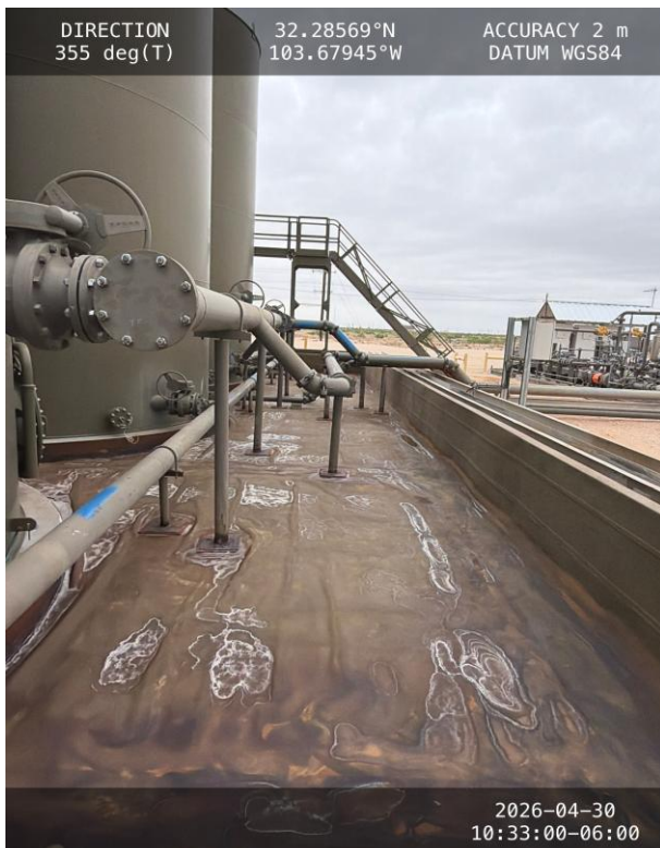
Photo 7 View of east side of containment towards north.
