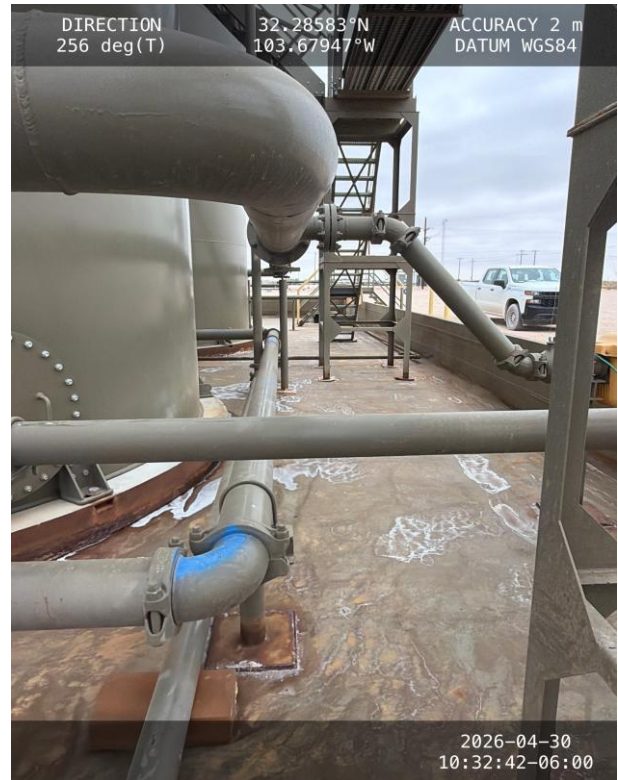
Photo 6 View of east side containment towards north.
