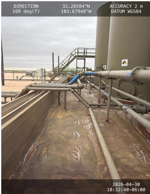
Photo 5 View of east side containment towards south.
