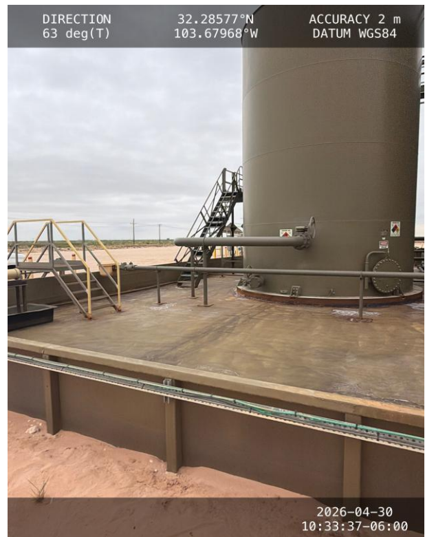
Photo 8 View of northwest corner of containment.
