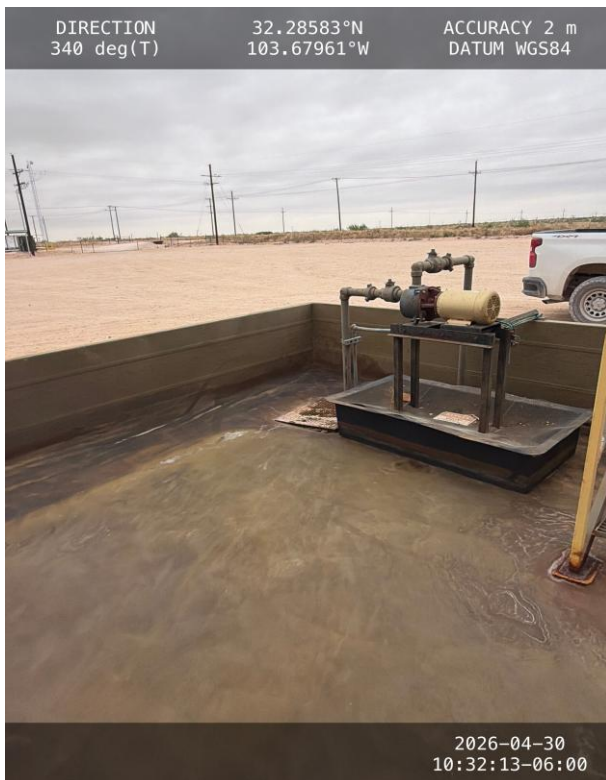
Photo 3 View of northwest corner of secondary containment.
