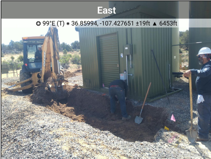
Photograph: 5 Date: 04/20/2026 Description: Hand digging around utilities north of pump shed View: East
