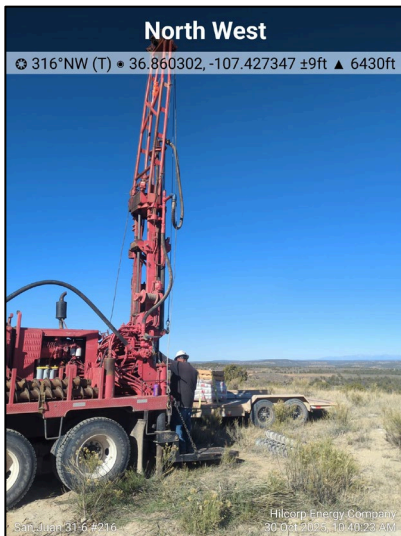
Photograph: 3 Date: 10/30/2025 Description: Conducting depth-to-water boring BH01 at Site View: Northwest
