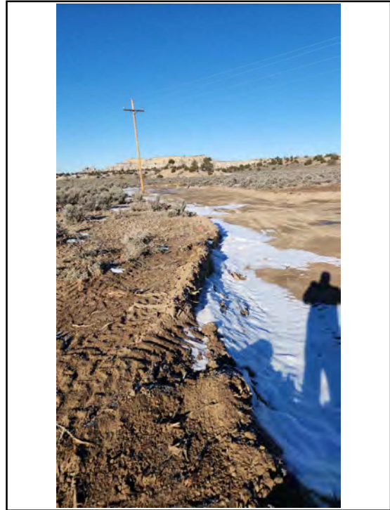
Photo 30 Looking northwest, overview of the excavation in the field.
