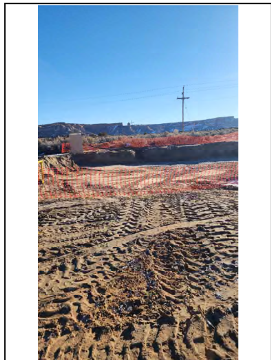
Photo 28 Looking east, overview of the northern section of the main excavation.
