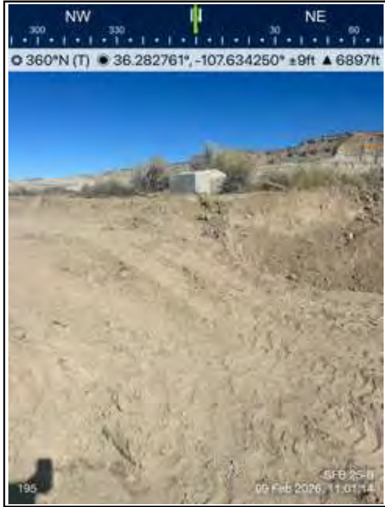
Photo 13 Looking north with secondary access ramp.
