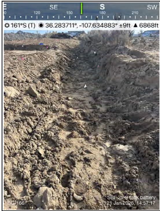
Photo 21 Excavation within the ditch along access roadway.
