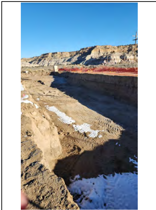
Photo 27 Looking northeast, overview of the main excavation area.
