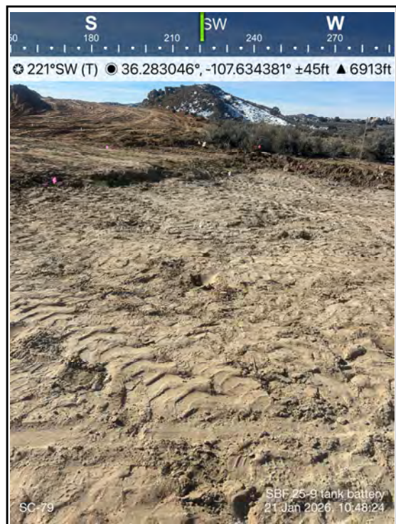
Photo 16 Area on the far north end of the facility.
