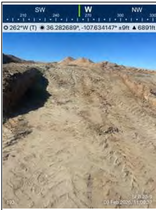
Photo 11 West wall continued on the main excavation and access ramp.
