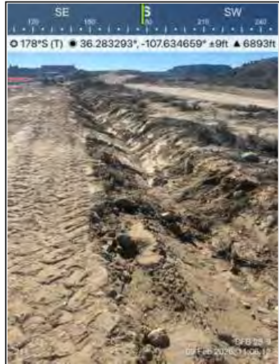
Photo 18 Excavation area in the access road.
