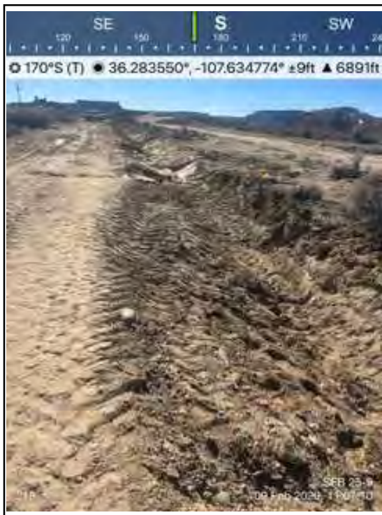
Photo 19 Excavation area in the ditch following the access road.
