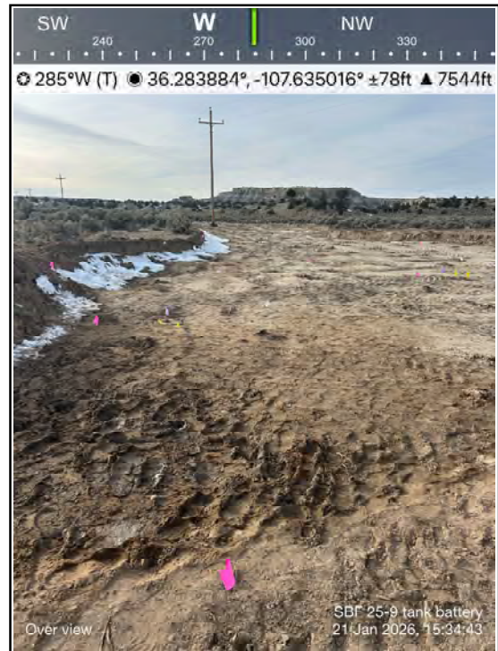
Photo 22 Excavation of the release area in the field.
