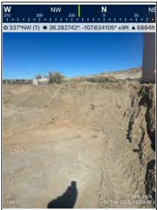
Photo 7 North wall on main excavation below the former tank battery.
