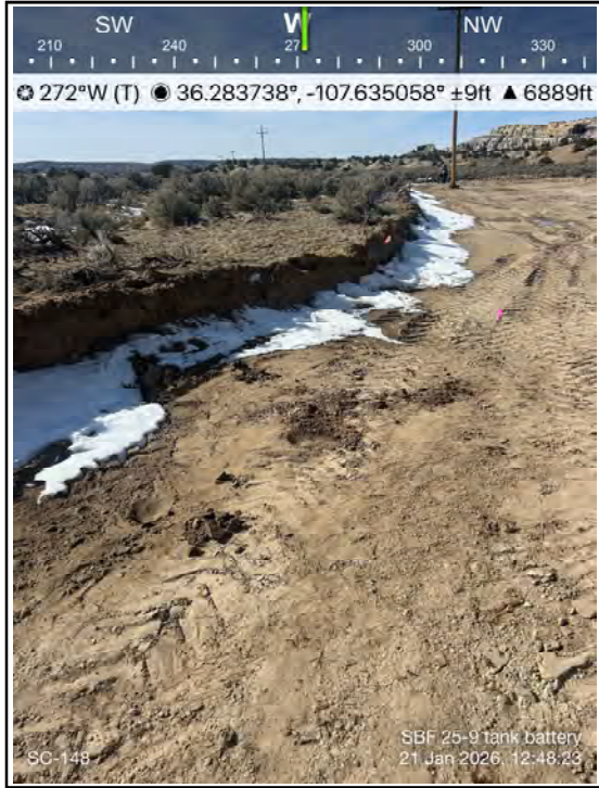
Photo 25 Excavation of the release area in the field.
