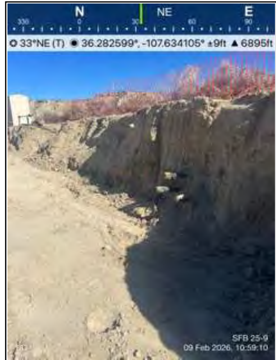
Photo 6 East wall continued on main excavation below the former tank battery.
