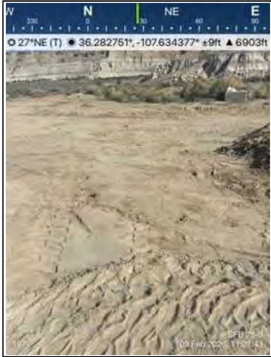
Photo 17 Excavation area in the access road.
