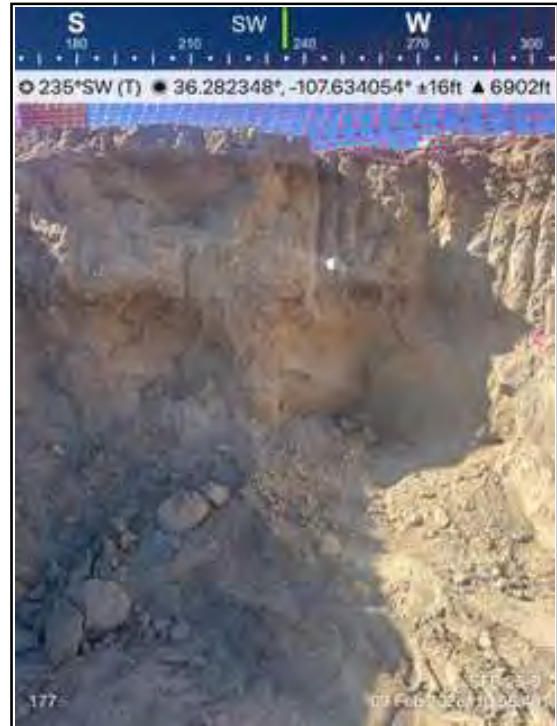
Photo 2 South wall and southwest corner of the main excavation below the former tank battery.
