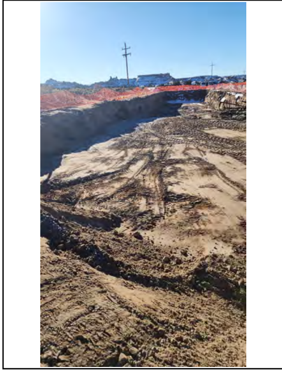
Photo 29 Looking south, overview of the main excavation.
