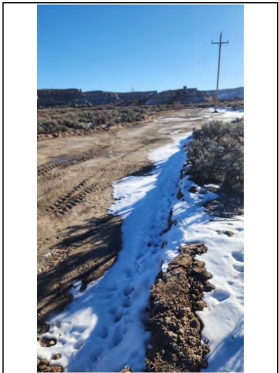
Photo 31 Looking southwest, overview of the excavation in the field.
