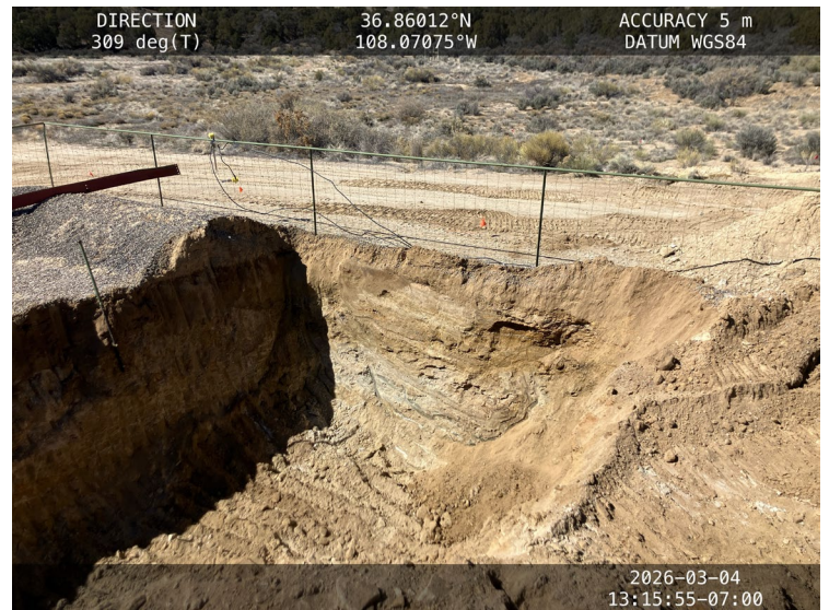
Photograph: 8 Date: 03/04/2026 Description: Final excavation extent View: Northwest
