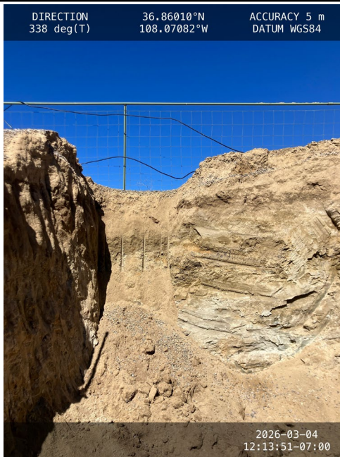
Photograph: 7 Date: 03/04/2026 Description: Excavation sidewall View: North
