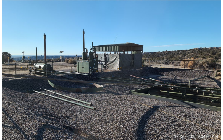
Photograph: 2 Date: 12/17/2025 Description: Release area and former AST location within secondary containment following tank removal. View: North
