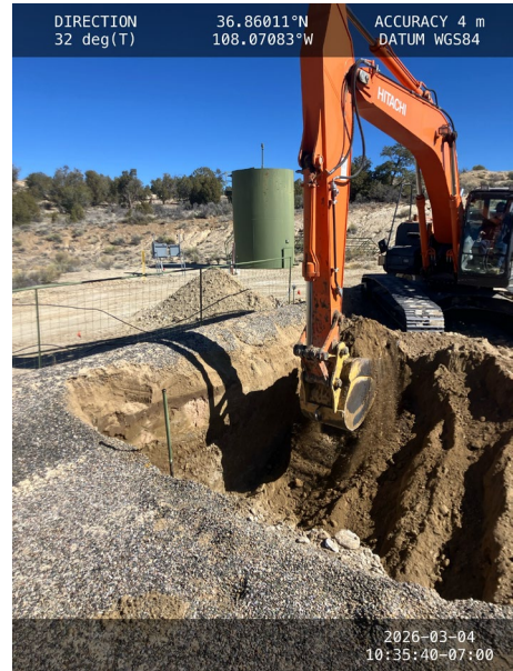
Photograph: 6 Date: 03/04/2026 Description: Excavation activities. View: North
