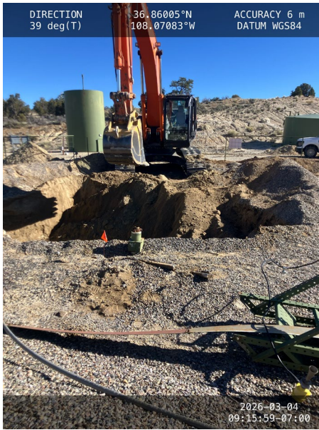
Photograph: 5 Date: 03/04/2026 Description: Excavation underneath bermed area View: North
