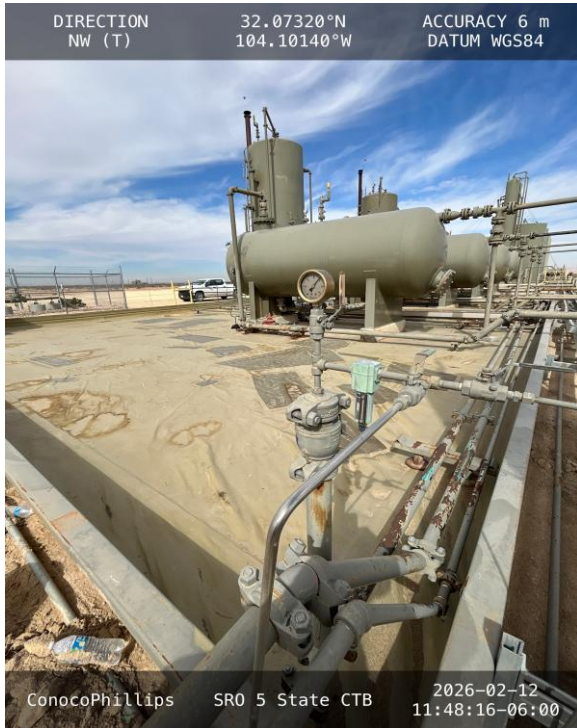
Photo 17 View of southeast corner of secondary containment.
