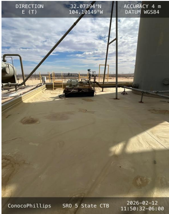
Photo 5 View of north side of secondary containment towards east.
