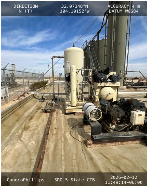
Photo 11 View of west side secondary containment towards north.
