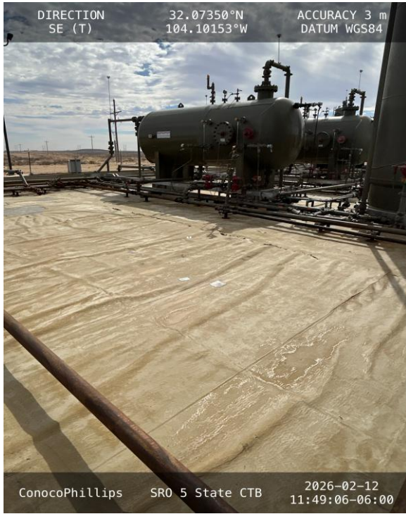
Photo 13 View of central portion of secondary containment towards southeast.
