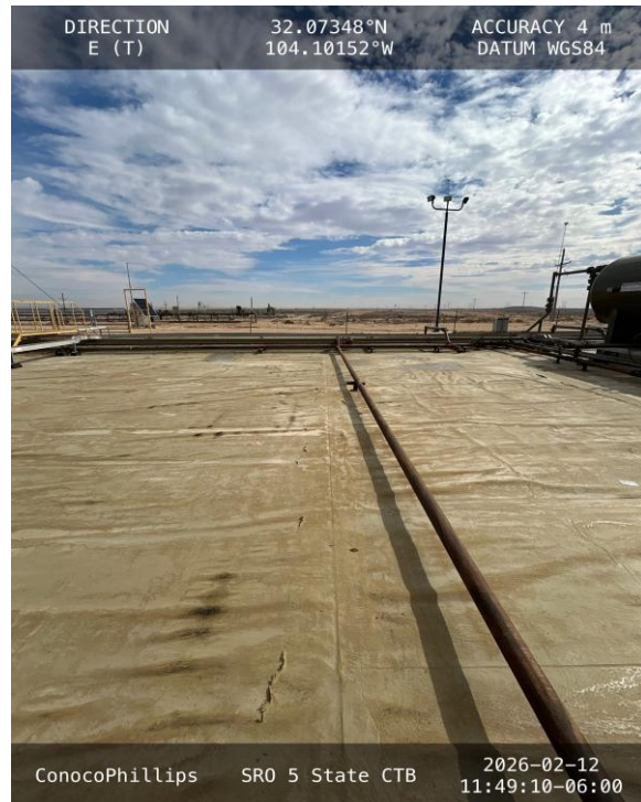
Photo 12 View of south side of secondary containment towards east.
