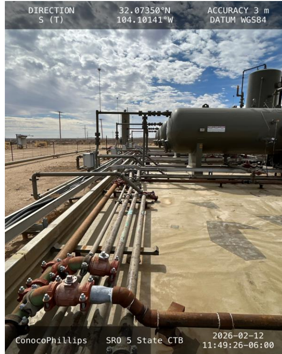
Photo 10 View of east side of secondary containment towards south.
