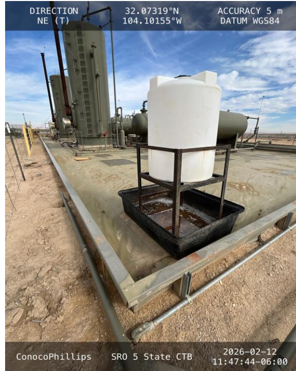
Photo 18 View of southwest corner of secondary containment.
