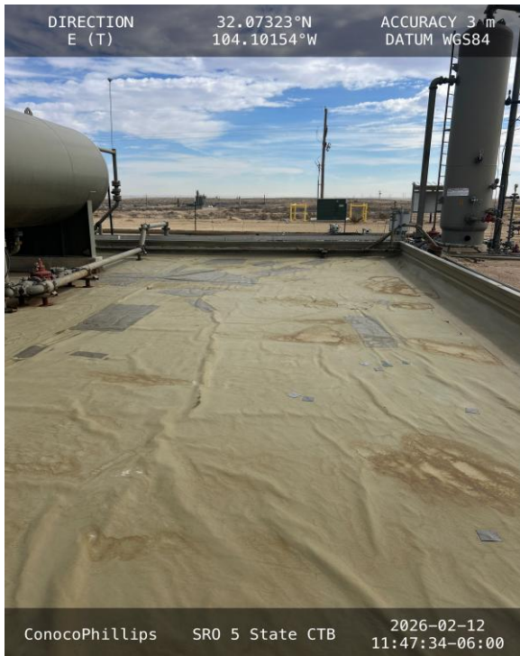
Photo 19 View of south side secondary containment towards east.
