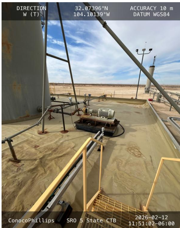
Photo 3 View of north side of secondary containment towards west.
