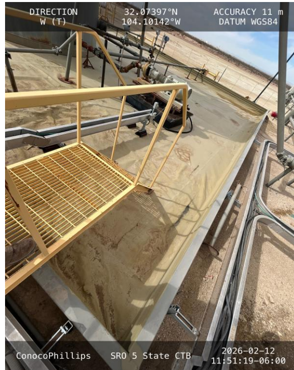
Photo 2 View of northeast corner of secondary containment.
