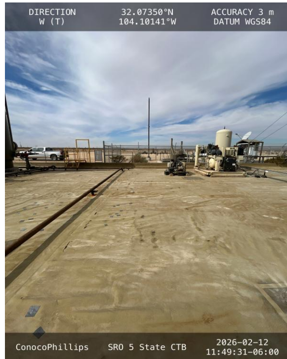
Photo 8 View of south central portion towards west.
