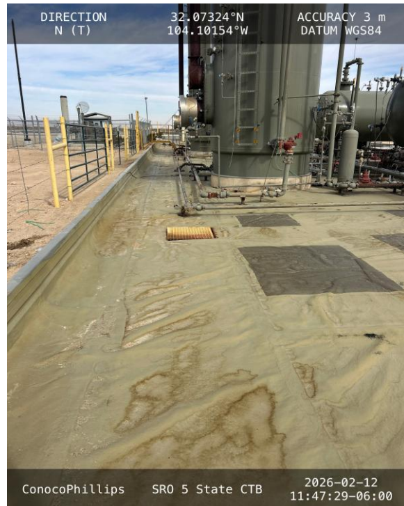
Photo 20 View of west side of secondary containment towards north.
