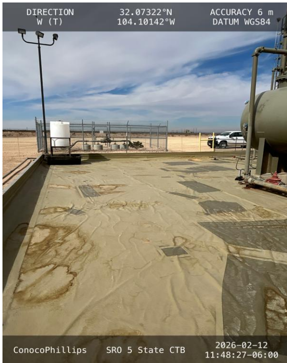
Photo 15 View of south side of secondary containment towards west.
