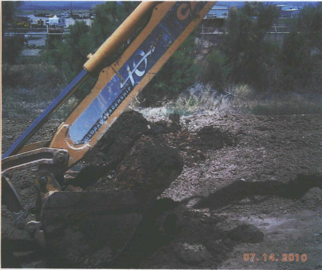
Below-Photo of Cell-2N-VZ-2 shows oily stained dirt about one foot under surface.
