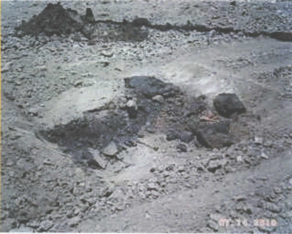
Below-Photo of Cell-2N-VZ-4 shows oily stained dirt about one foot under surface.
