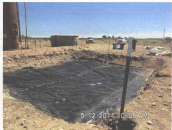
30x40 ft, 20-mil, reinforced liner installed at 4 ft
