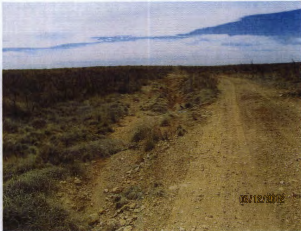
3. Drainage 1 - Downstream Viewing Southwest, March 12, 2012
