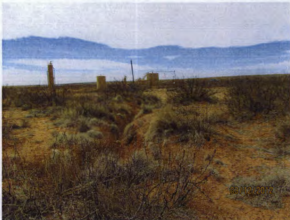
10. Drainage 3 – Termination Viewing Southwest, March 12, 2012
