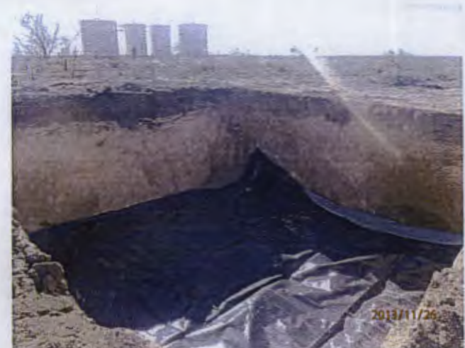
Installed 30'x30', 20-mil poly liner at 11.5', facing southwest
