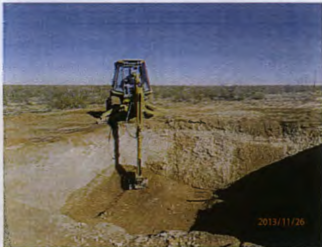
Installed 6" pad above liner, facing northeast 11/20/13
