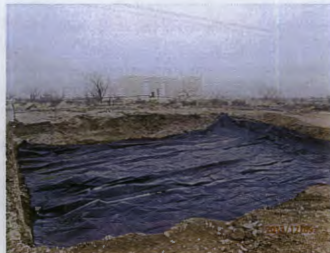
Installed 35'x40', 20-mil poly liner at 4.5 ft bgs, facing southwest 12/9/13
