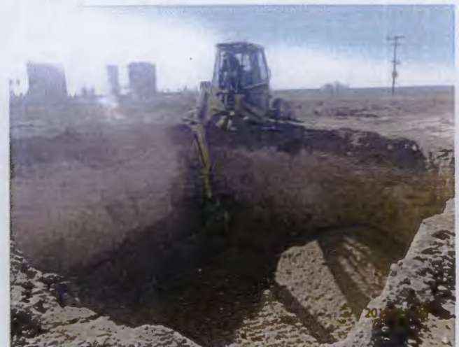
Installing 6" sand pad at base of excavation, facing southwest
