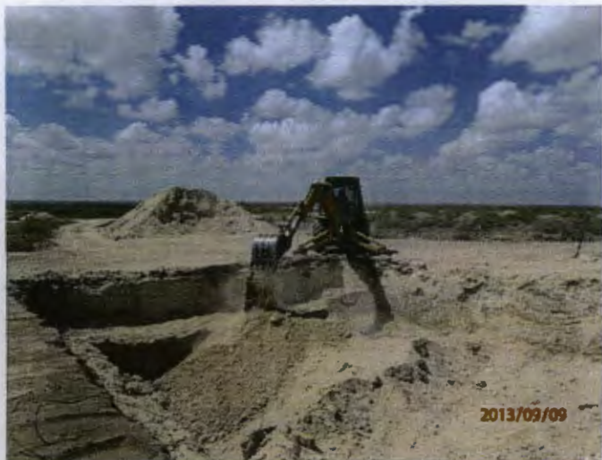
Backfilling excavation to 5' BGS, facing northwest 9.9.13
