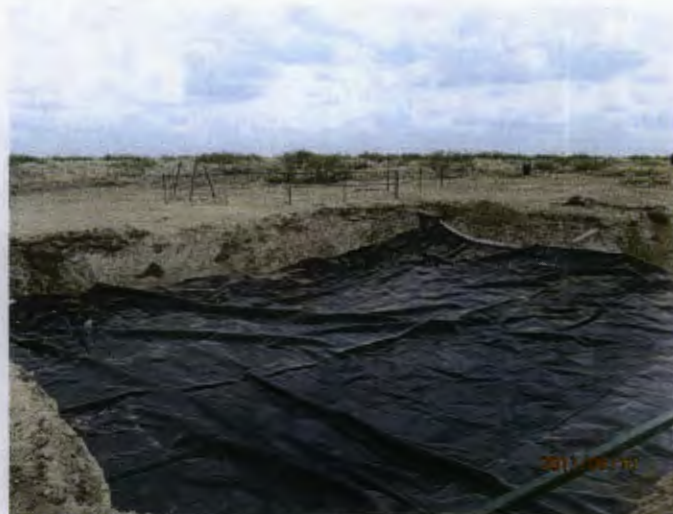
Installed 40'x 35', 20'mil reinforced liner, facing northeast 9.10.13
