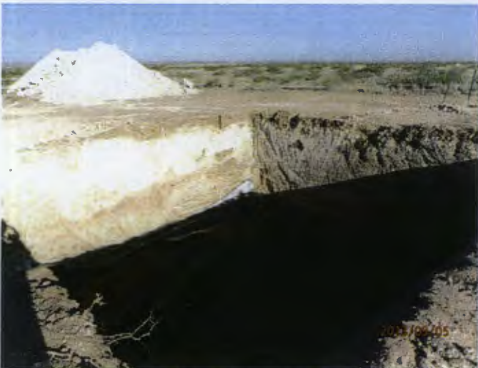
Installed 30'x 30', 20-mil reinforced liner, facing northwest 9.5.13
