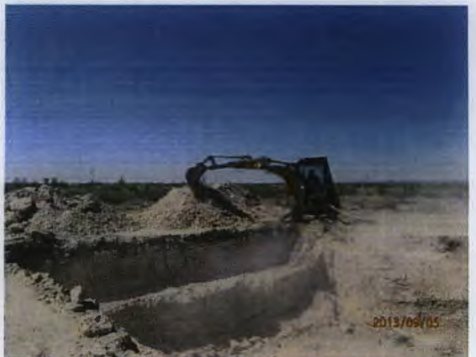
Benching excavation, facing southwest 9.5.13
