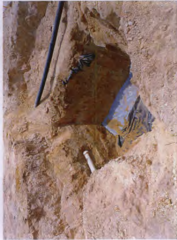
Installing 10'x5', 20-mil poly liner at 12' bgs, facing northeast
