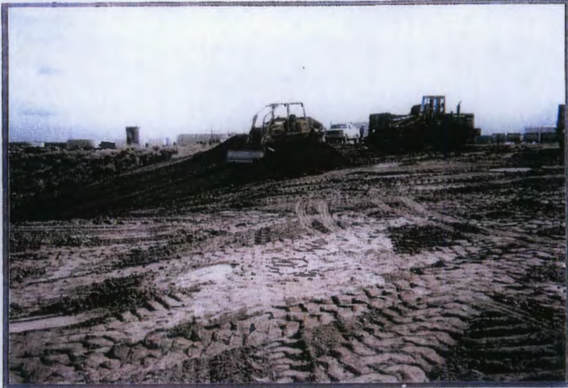
Side Slope Construction
