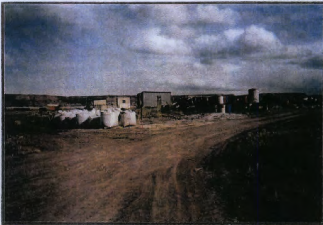
View of Adjacent Equipment Laydown Area
