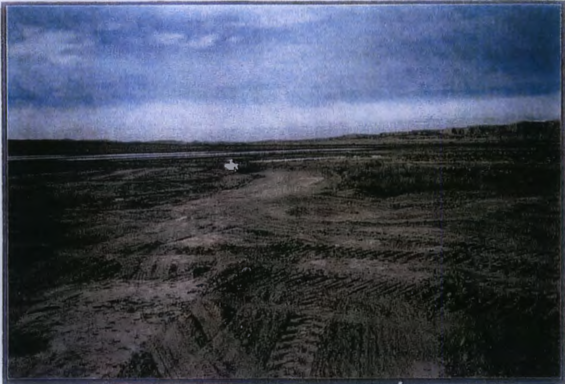
Access Road Being Removed From Site
