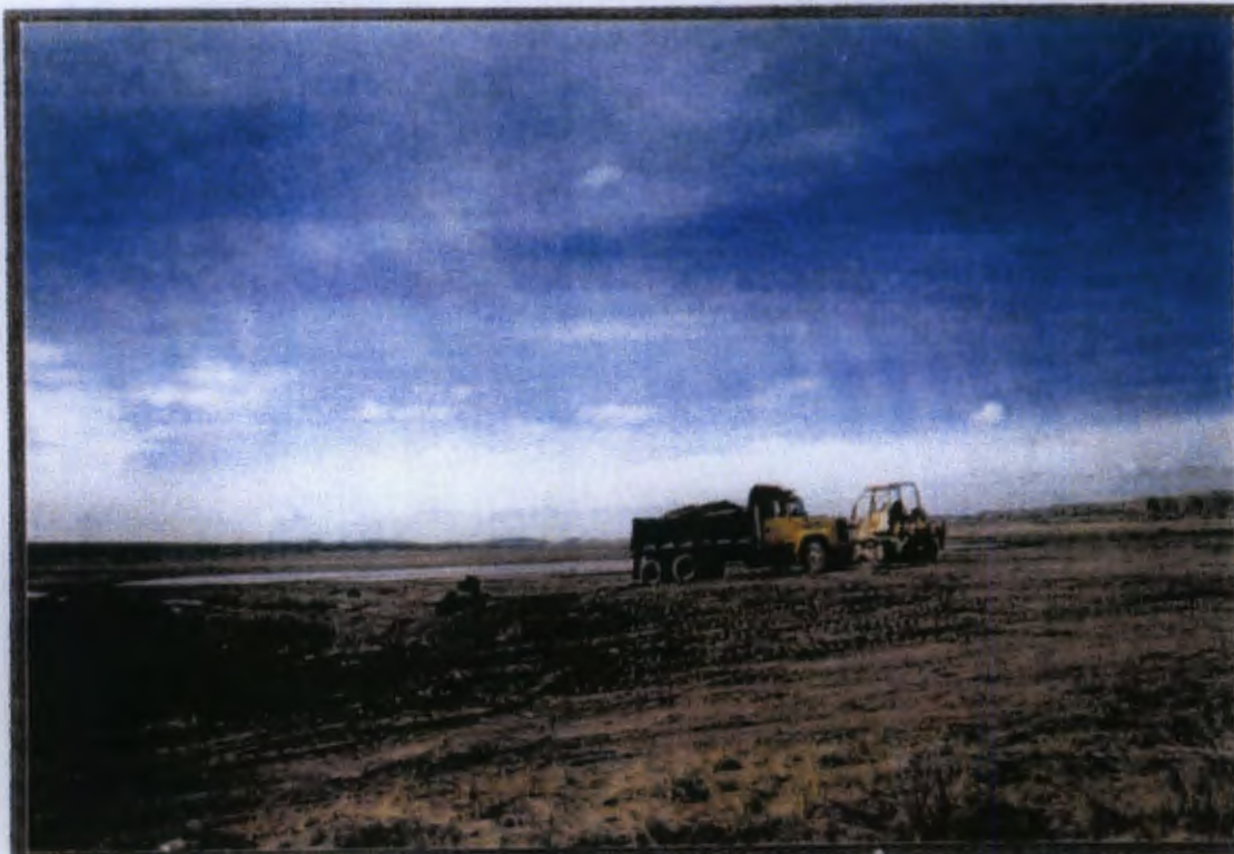
Clean Soil Being Trucked To Site
