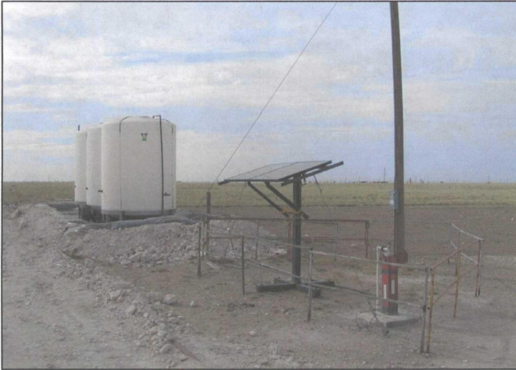
**Figure 9** – Groundwater recovery well (RW-1) installed at Vacuum K-35-1 boot. The groundwater pump in this well is powered by solar-generated electricity. Recovered groundwater is stored in temporary tankage and subsequently used for SWD system maintenance.
