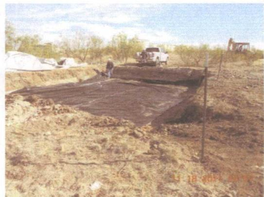
36x31-ft, 20-mil reinforced liner installed, facing northeast
