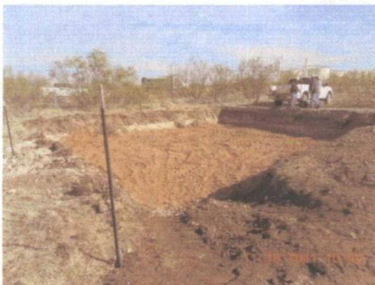
36x31x5-ft bgs excavation complete, with 6" blow sand pad, facing northeast
