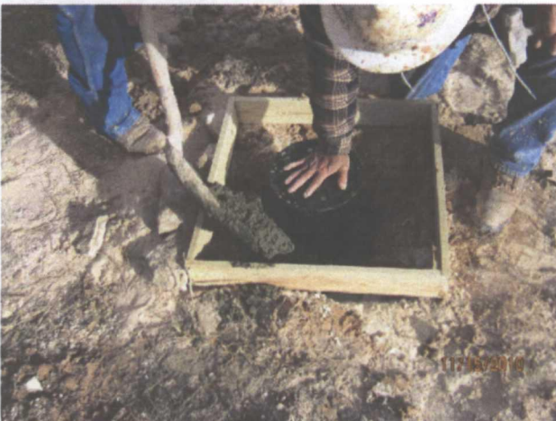
Concreting the flush mount
