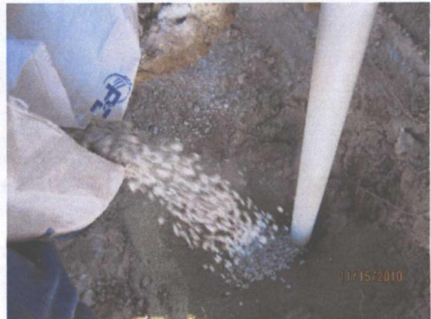
Adding the bentonite seal
