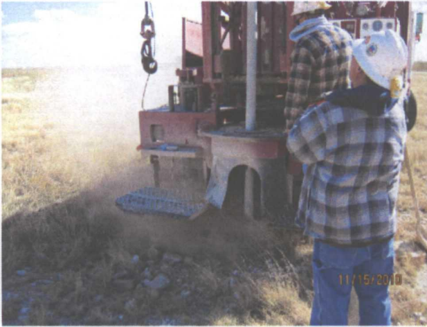
Drilling the monitor well
