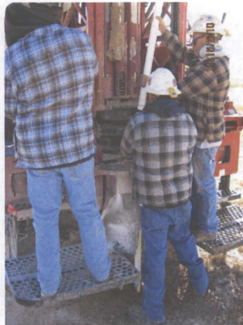
Inserting the casing
