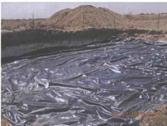
Plastic liner installed over pad, facing southwest 9/22/11
