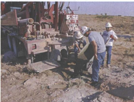
Plugging the bore with a 1- 3% bentonite/concrete slurry, facing north 9/1/11
