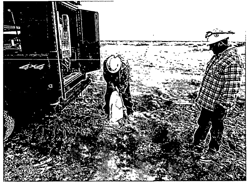
Plugging Pt. 3 bore in total with bentonite
