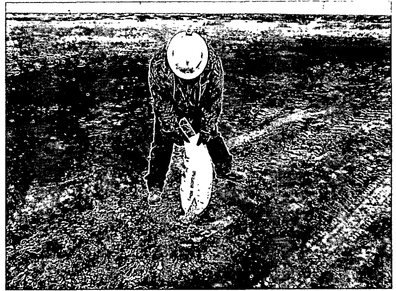
Plugging Pt. 5 bore in total with bentonite
