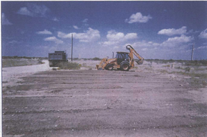
spreading clean, imported soil on surface
