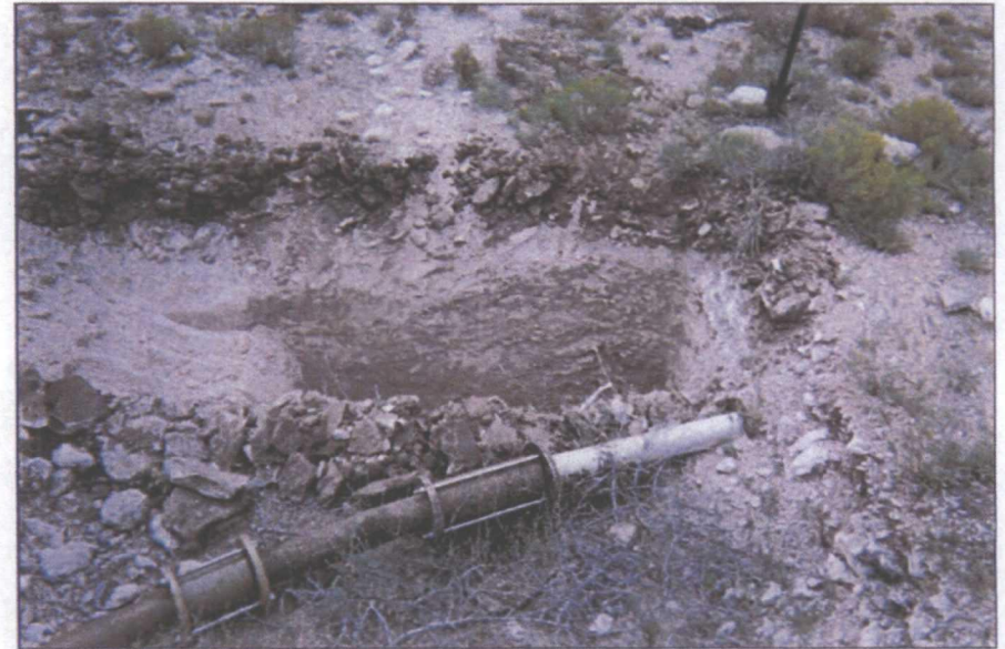
6-ft-deep delineation trench at former box site
