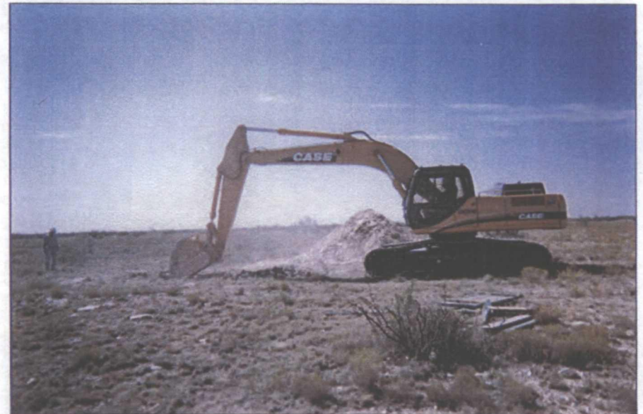
box removed; delineation and excavation
