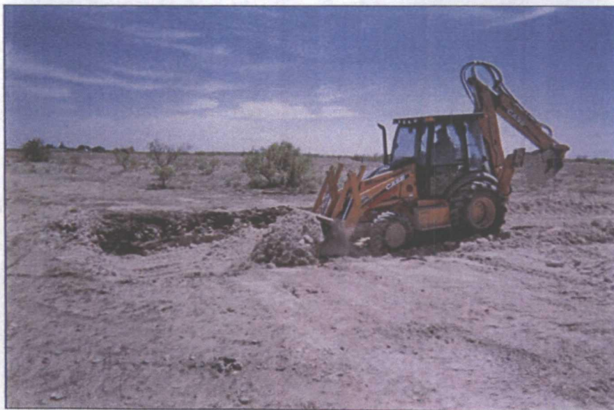
backfilling 20 x 15 x 12-ft excavation
