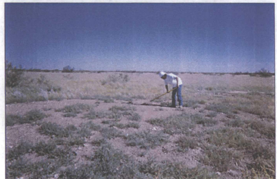
seeding disturbed area of backfilled site
