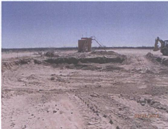
Backfilling with imported caliche up to 4' BGS,
