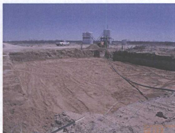
Installed bottom 6'' blow sand pad, facing
