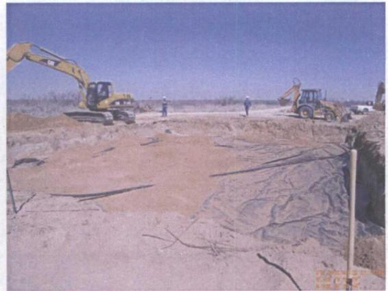
Installing top 6" blow sand pad above liner,
