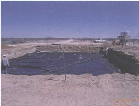
Installing 62 x 51 ft 20-mil reinforced liner,
