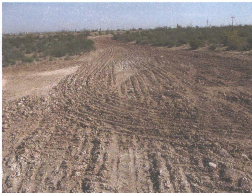
Photograph 23. South Pit Area After Grading and Ripping
