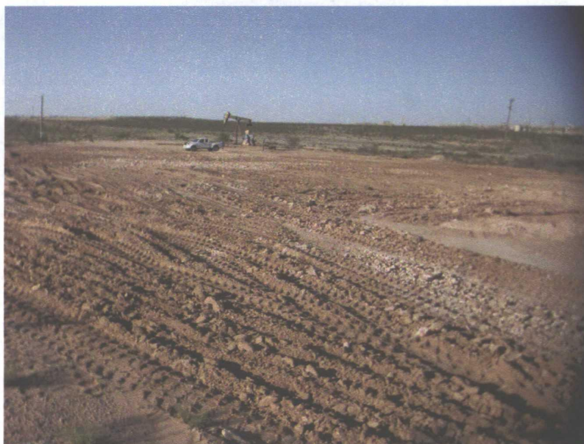
Photograph 24. South Pit Area After Grading and Ripping
