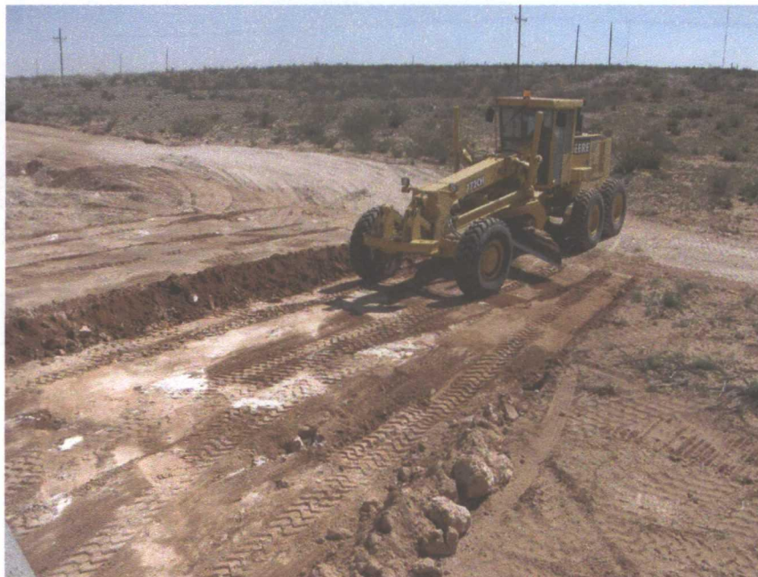
Photograph 11. Excavating the Top Foot of Chloride-Stained Soil Near the North Pit
