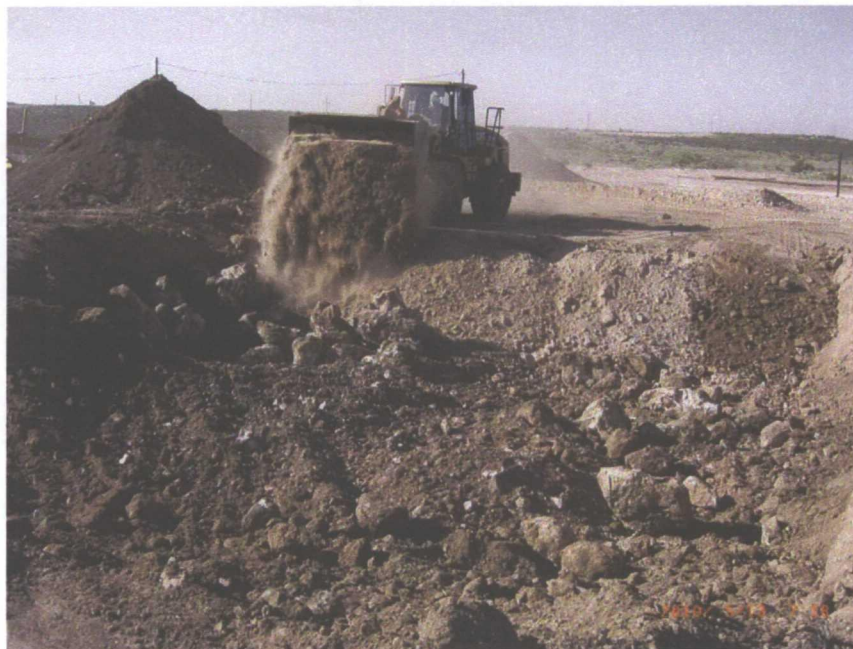
Photograph 15. Backfilling the South Pit excavation
