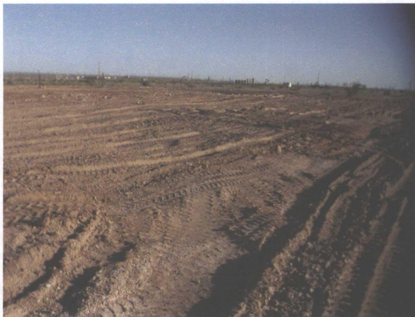
Photograph 25. North Pad After Grading and Ripping
