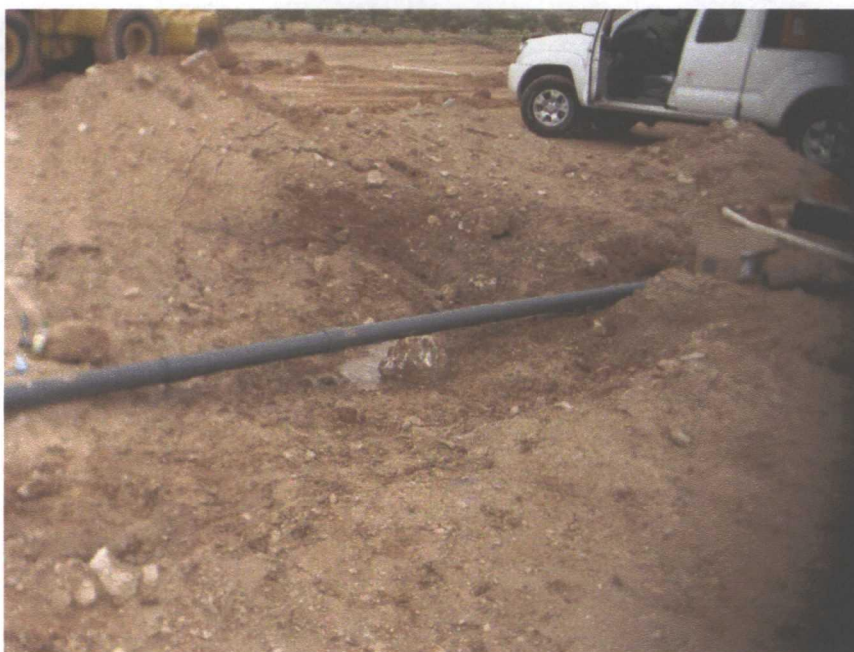
Photograph 22. Replaced Broken PVC Pipe Within the North Pit
