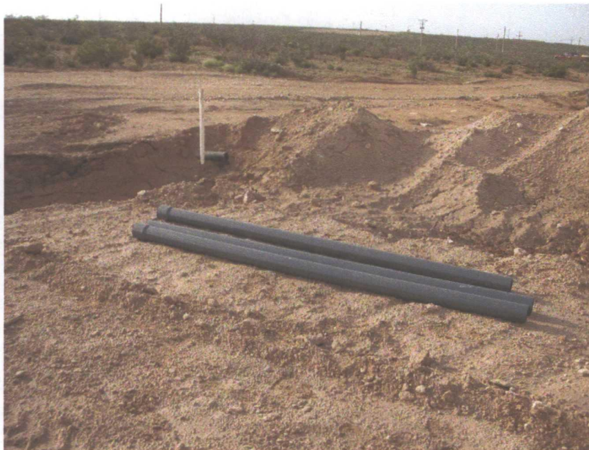
Photograph 21. Replacing a Broken PVC Pipe Within the North Pit
