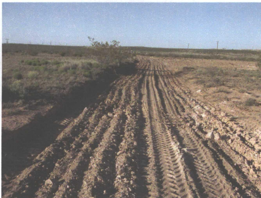
Photograph 26. Graded and Ripped Access Road
