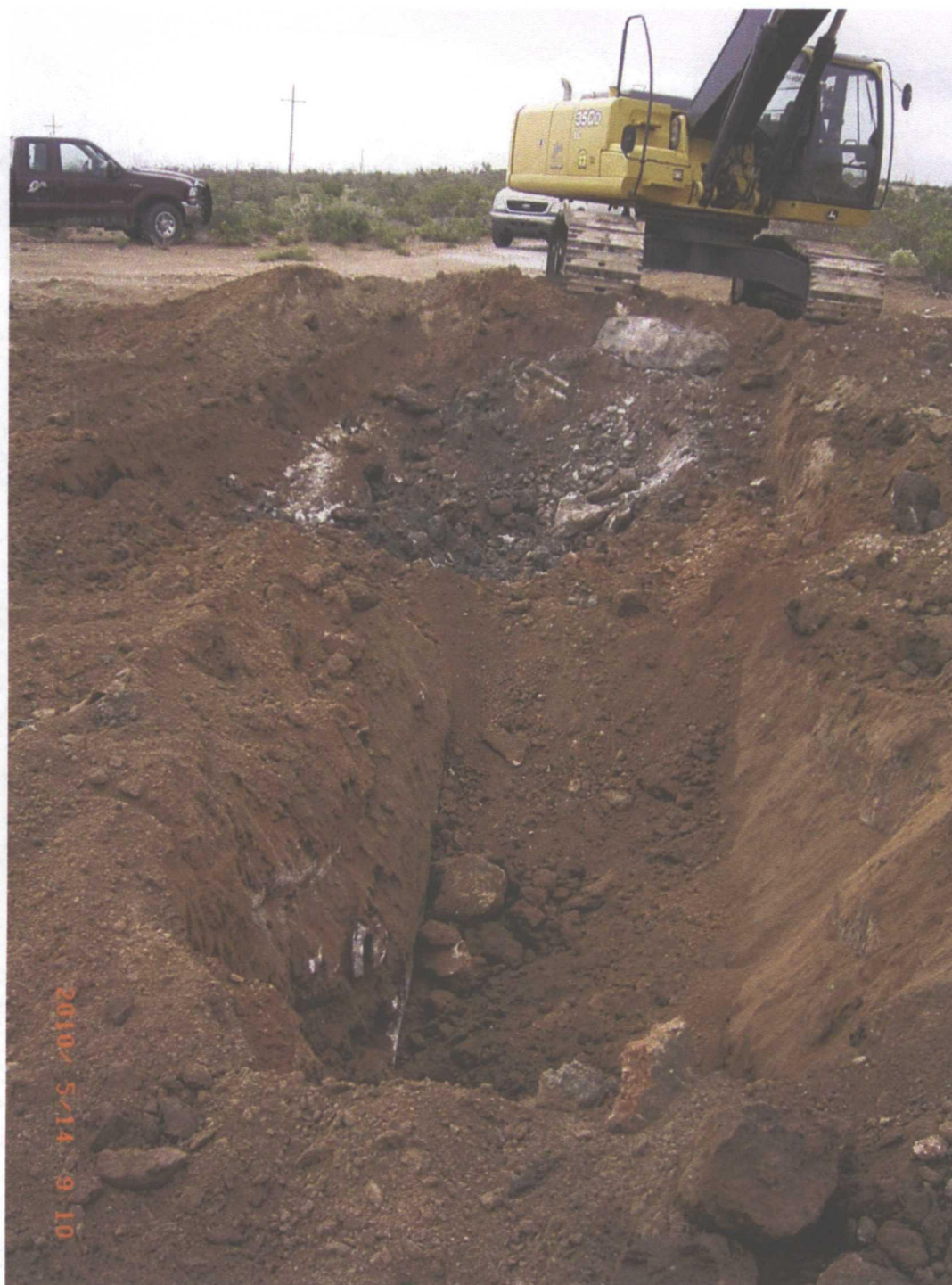
Photograph 18. Excavating the Extent of Hydrocarbon Contamination of the Former Tank Battery
