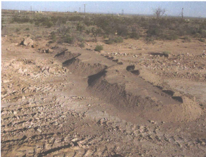
Photograph 30. A Berm Near the South Pit to Prevent Surface Runoff
