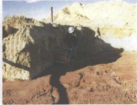
Compacting existing clay layer and installed clay layer edges 10/30/07
