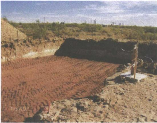
Installed clay layer to extended 75' x 45' area at 6' bgs 10/29/07
