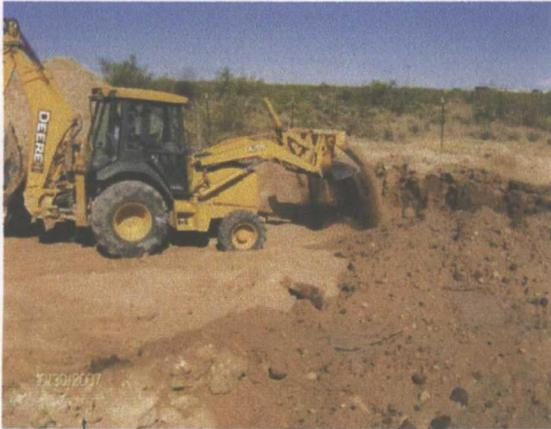
Backfilling excavation up to 1' bgs 10/30/07
