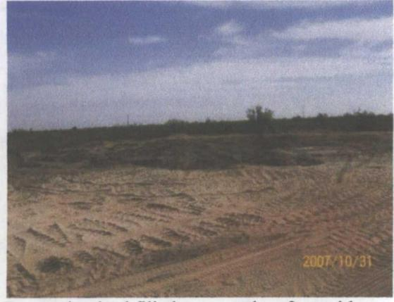
Excavation backfilled to ground surface with clean soil and amendments 10/31/07
