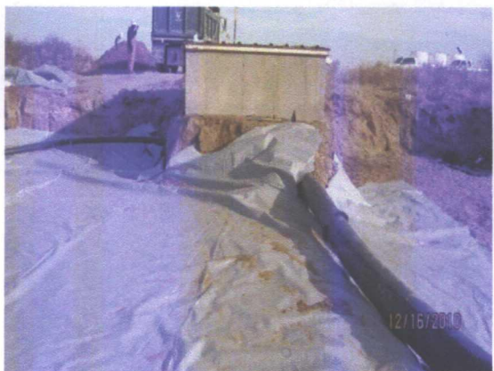
installing the plastic liner
