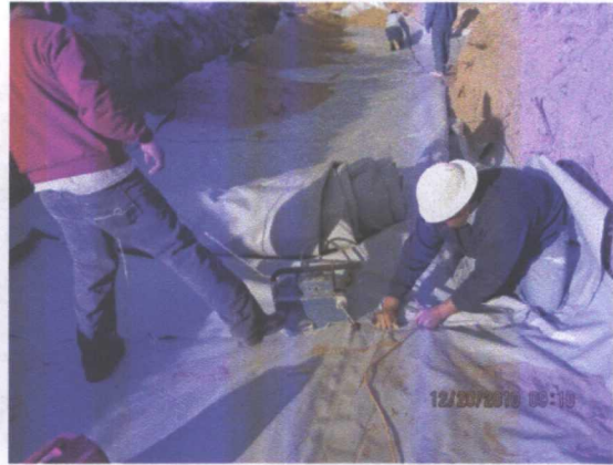
seaming the liners together
