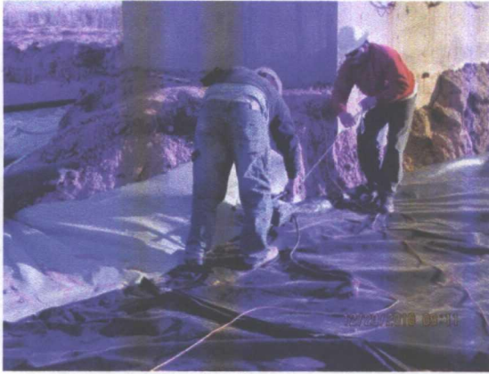
seaming the liners together
