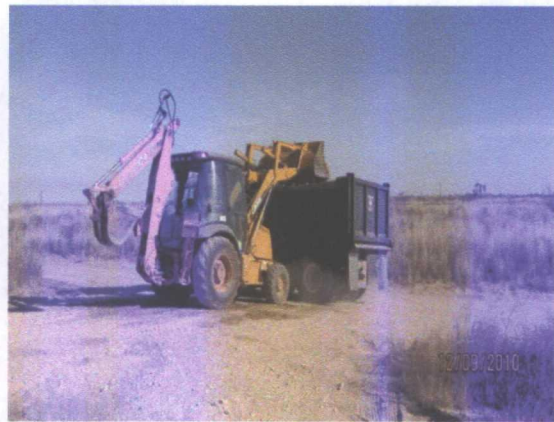
hauling excavated soil to Sundance for disposal
