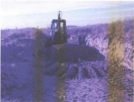
excavating the site
