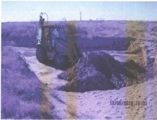
excavating the site
