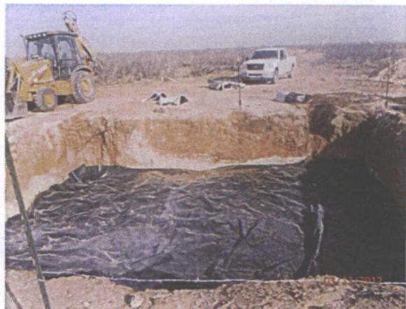
Installed 30'x25' 20 mil reinforced liner, facing northwest 3/13/2012
