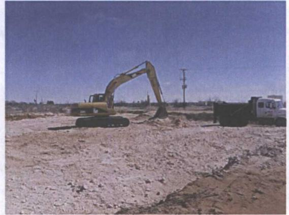
backfilling with caliche, facing south 2/27/2013
