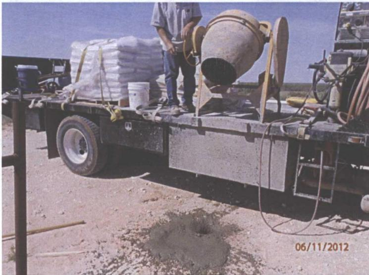
Installing the 3 ft concrete cap, facing SW
