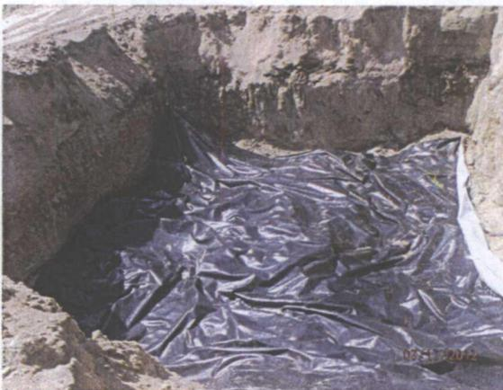
Installing 30'x30'x12' liner @ 12' bgs
