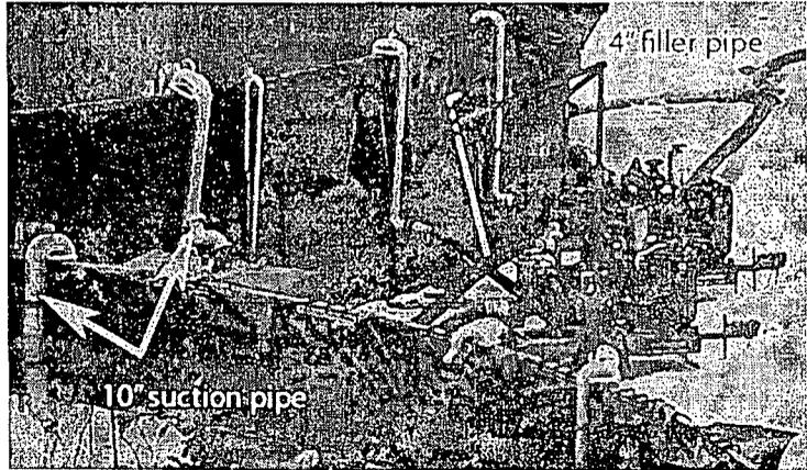
Photo 7: Photograph of the suction and filler pipes.
