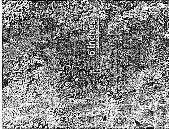
Photo 2: 6-inch caliche pad thickness. Dense clay underlies the pad.
