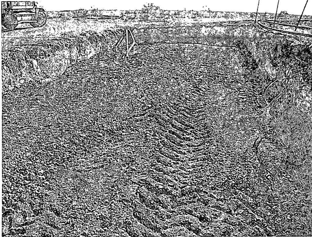
Clay liner installed in area of AH-1
