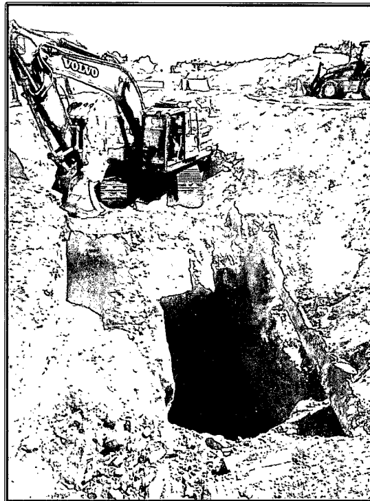
Photo 10: Final excavation depth of the Lateral C-7 Pipeline at 33.5' below ground surface along County Road 7007.
