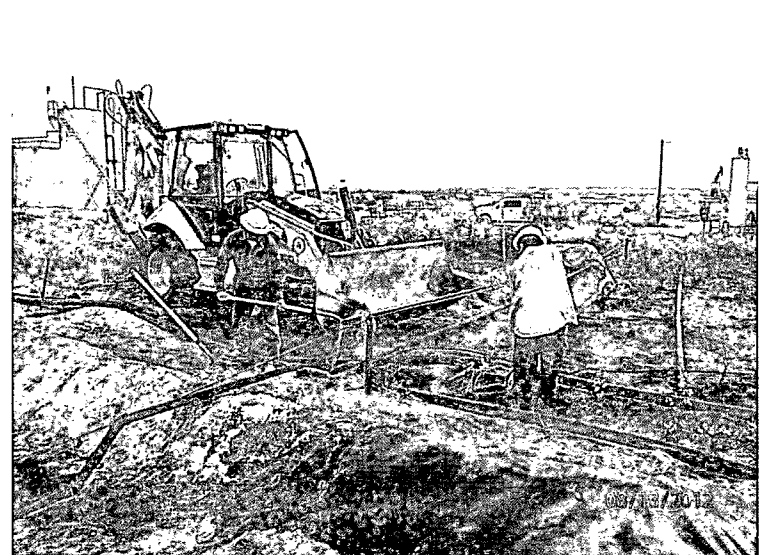
Excavating near lines, facing east
