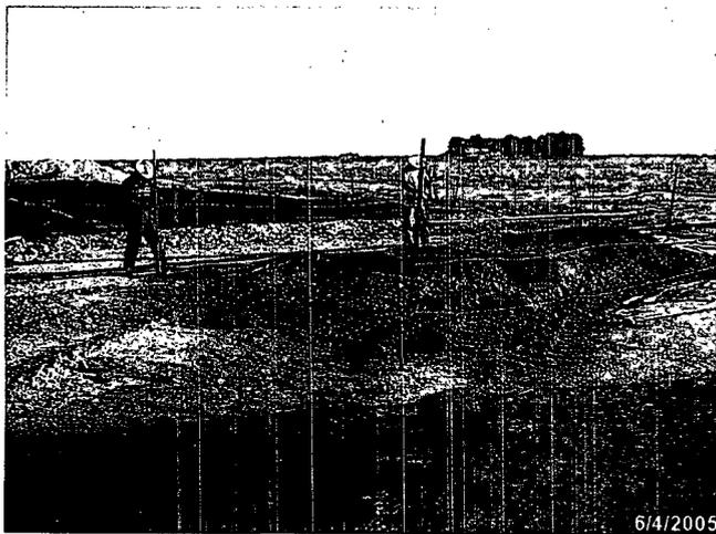
Photo #5: Excavated, diesel soaked soil stockpiled on plastic. Drilling pit is in background of photo.
