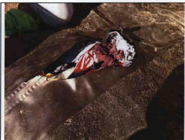
4.) Discovery of tear north of sump. Rags used to hold up liner during remaining cleaning activities.
