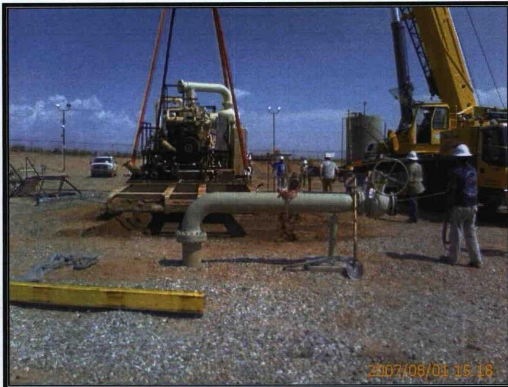
**Photo 1: Removing Compressor from Pad #1**
