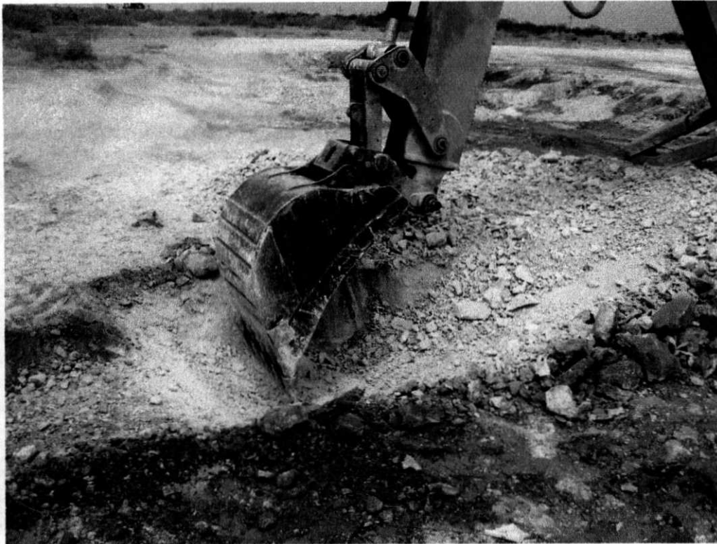
Photo 3. View of the backhoe trench being installed.
