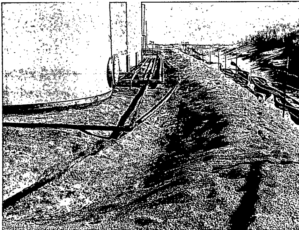
Back side of battery – Near AH-6
