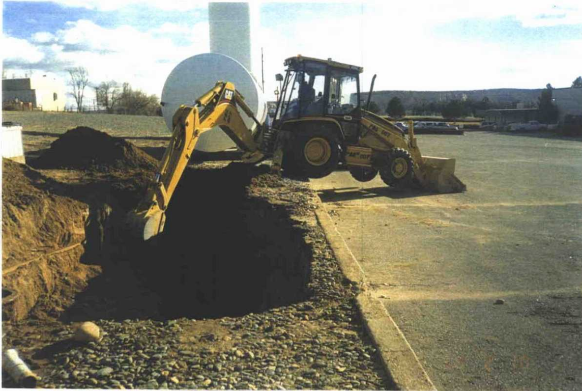
Photograph #1 Uncovering the AWT
