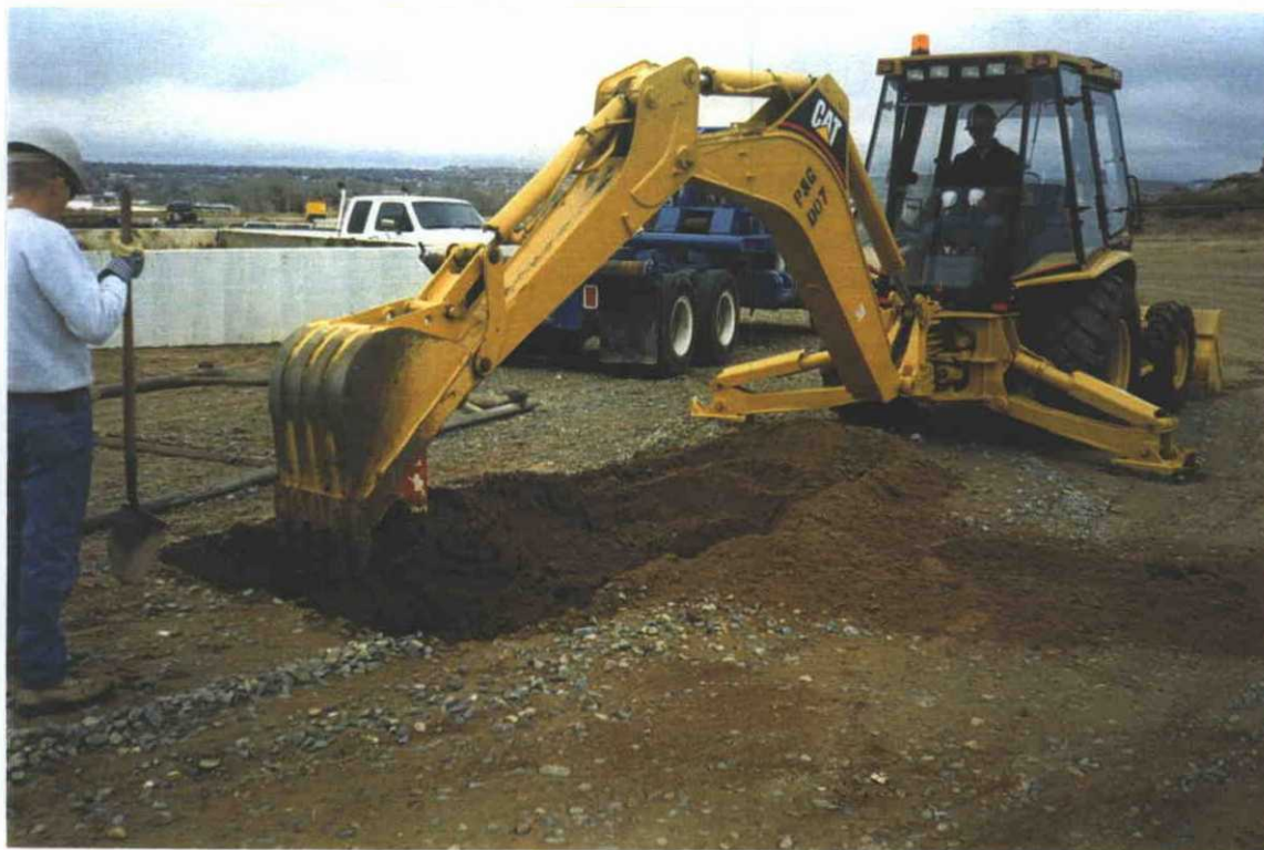
Photograph #6 Starting to Dig on the FWT
