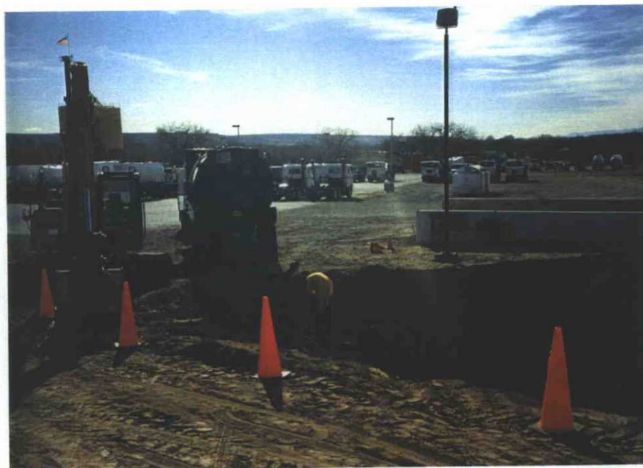
Photograph #12 Cleaning Sludge out of FWT
