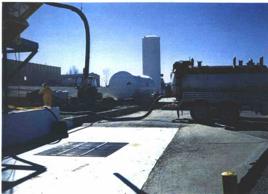
Photograph #2 Cleaning out the AWT Solids
