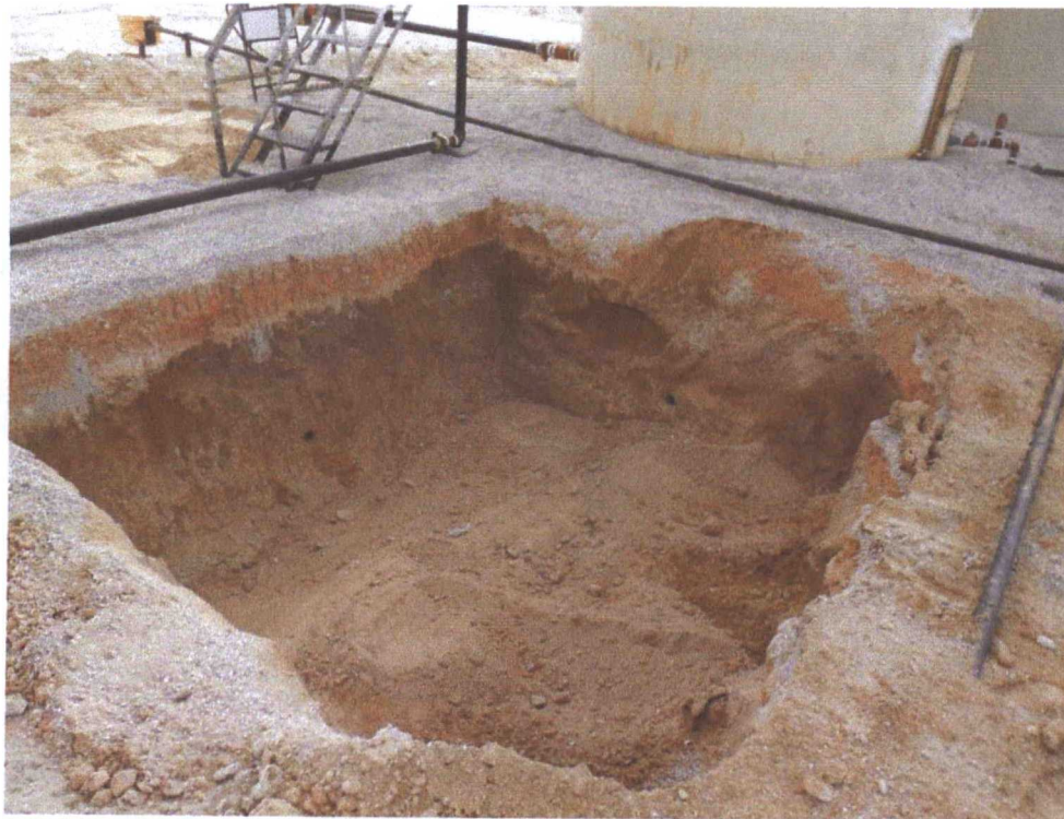
View South – AH-1 excavation area
